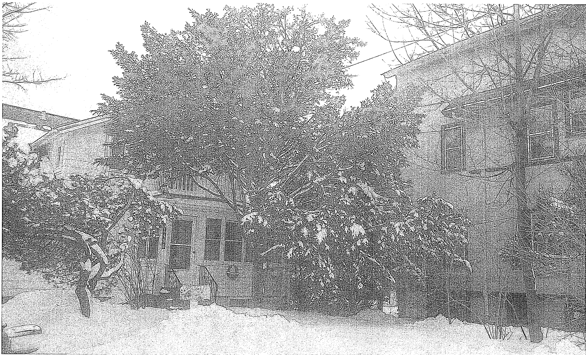
1435 MORRISON ST. (HOUSE TO THE WEST.)
