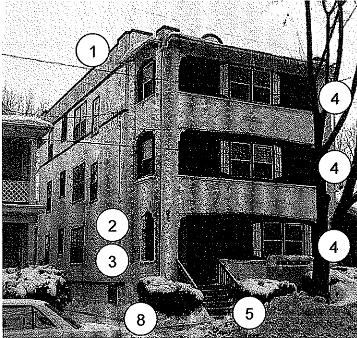
Northwest and Southwest Elevations (Front)
