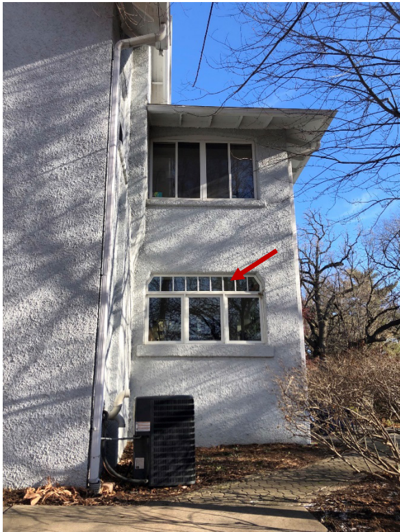
Photos showing the transom windows (red arrows) on the rear (south) and side (west) elevations of the house. The shed will have rectangular divided windows to match (see 3D rendering on previous page).
