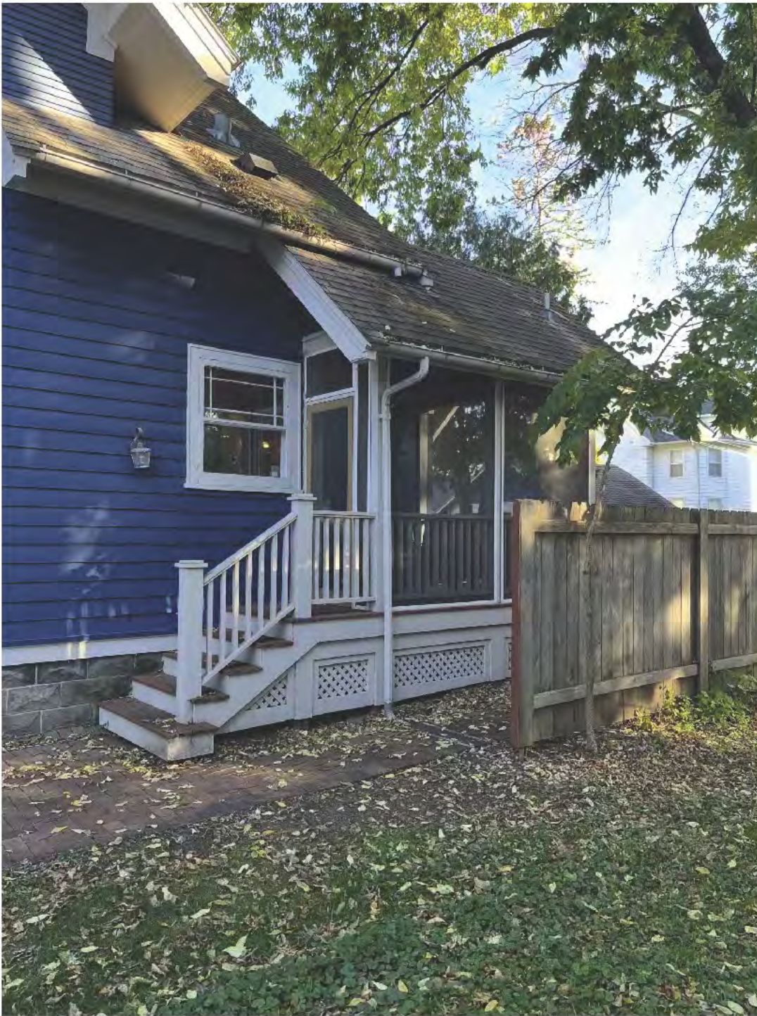
1717 Chadbourne Project Photos West Facade at Rear Screen Porch
