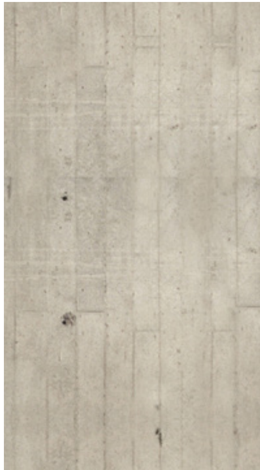
BOARD FORMED CONCRETE
