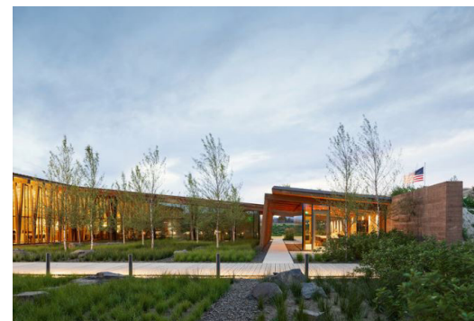
Continuity of Glulam structural system between columns and beams, with glass and concrete facade palette
