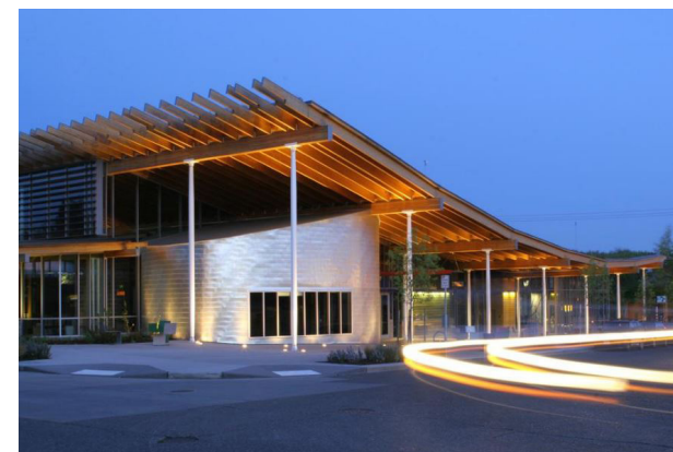
Glulam roof beams supported by steel columns
