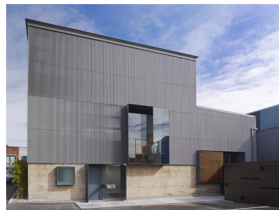
Perforated, corrugated metal facade by day
