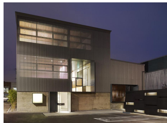
Perforated, corrugated metal facade by night
