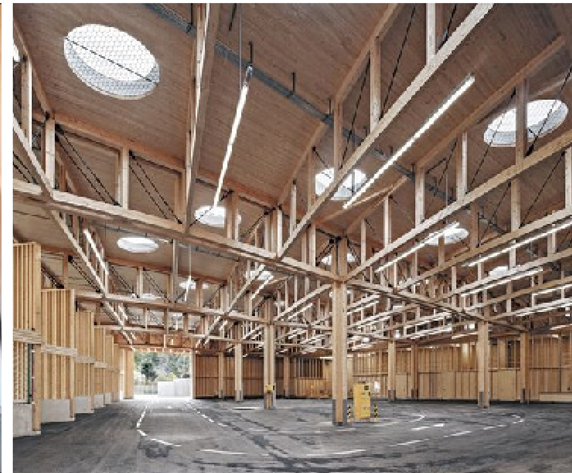
Large, open, light filled volume with a simple palette of materials
