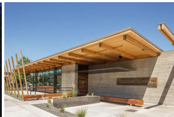
Material palette of boardform concrete and glass facade w/ glulam wood supported roof
