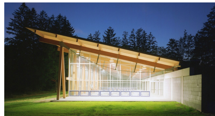
Glulam columns, beams and roof projecting over glass
