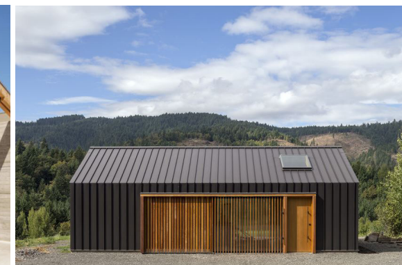
Metal roofing folds down to form walls
