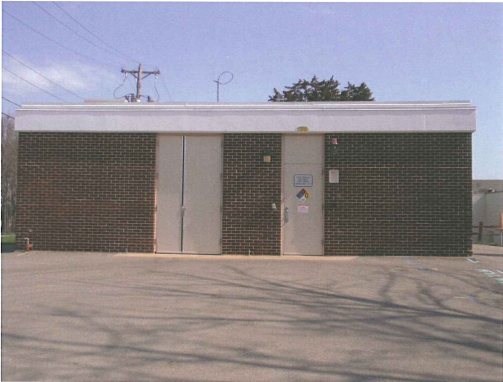
Picture 1 Southwest Elevation of Existing Pumping Station
