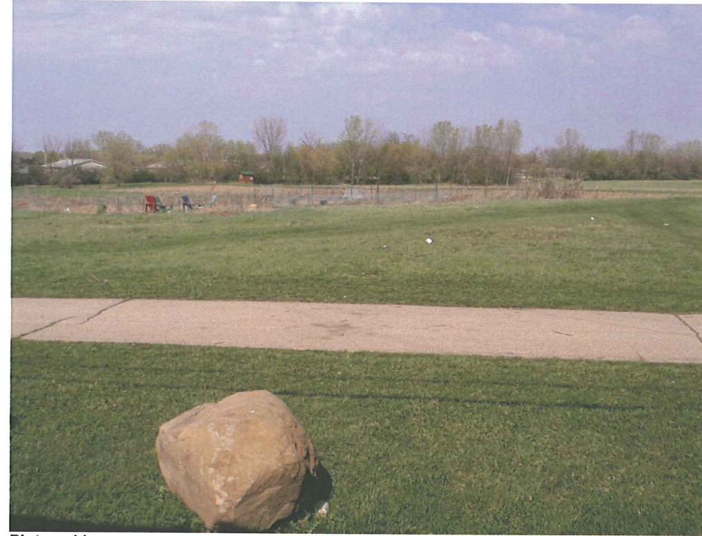
Picture 11 Facing northwest at northwest wall of existing pump station. Bike path, community garden, and Reindahl Park.
