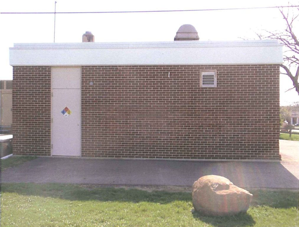
Picture 2 Northwest Elevation of Existing Pumping Station.
