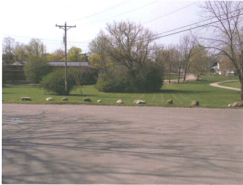
Picture 5 Facing southwest at southwest wall of existing pump station.
