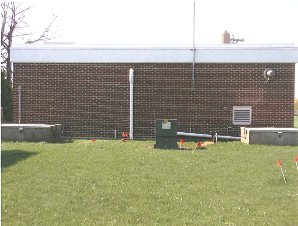
Picture 3 Northeast Elevation of Existing Pumping Station.
