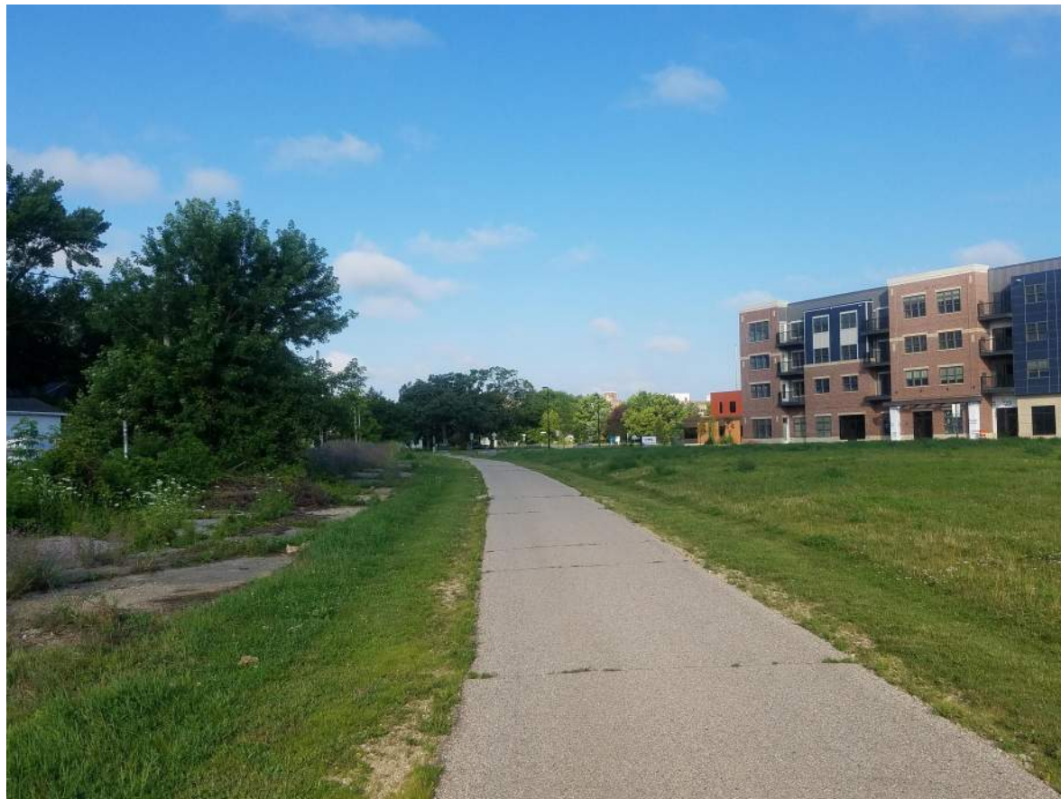
BIKE PATH LOOKING WEST - MIDDLE OF SITE
