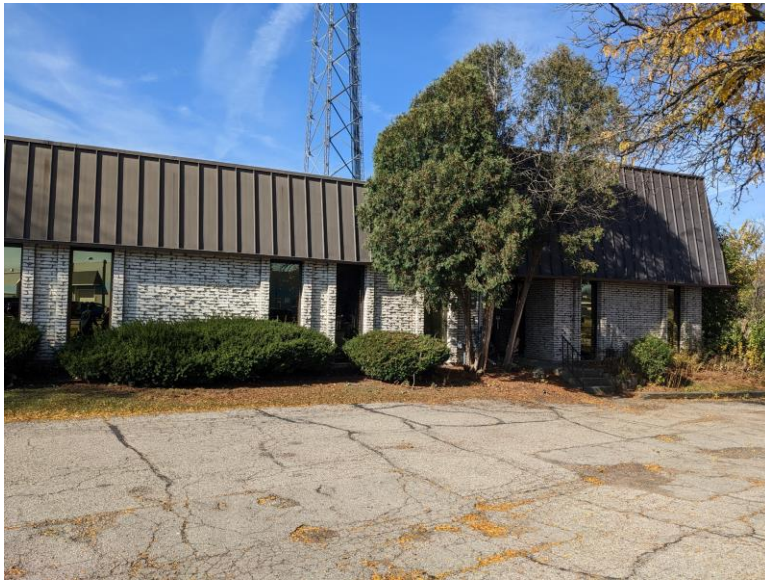
Photo 3: Front of building, parking lot
