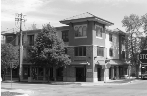
Figure D1: Entrance Orientation
