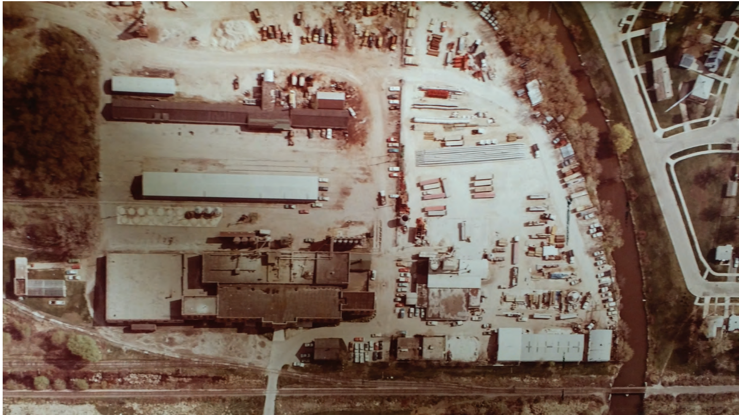
Aerial view of the Garver site, seen from directly overhead
