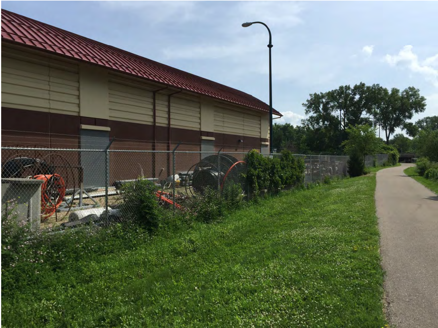
Traffic Engineering Yard M-10: Drainage Way
