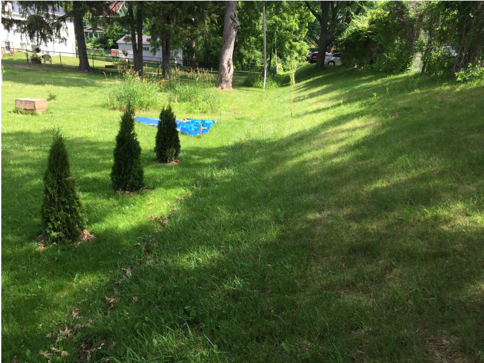
Traffic Engineering Yard M-5 : Drainage Way
