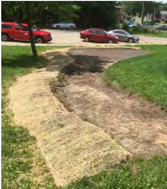
Photo on the left shows a rain garden that has been excavated and is ready for planting. The excavated soil was mounded on the downslope side of the hill to capture potential overflow.
