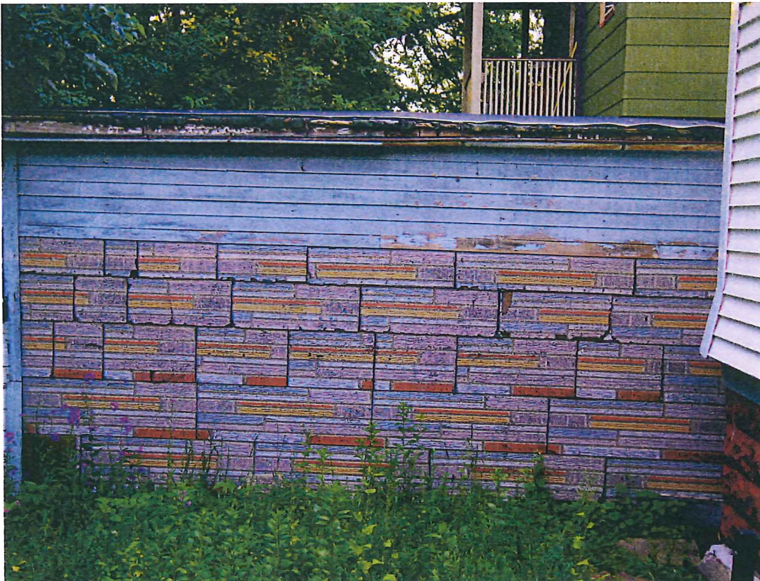
South side of garage
