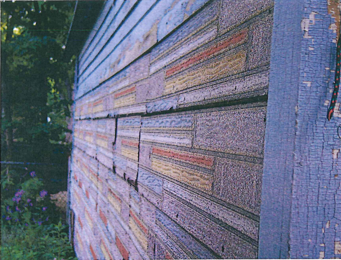
South side of garage
