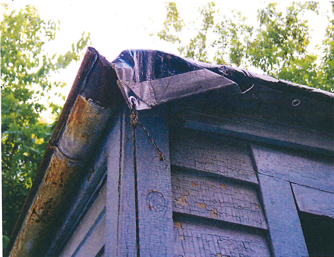
Tarpaulin on roof
