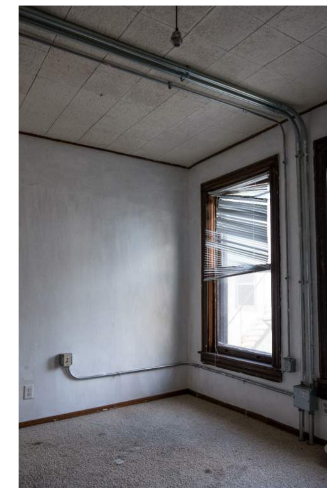
619 Lake Street - Interior No. 15
