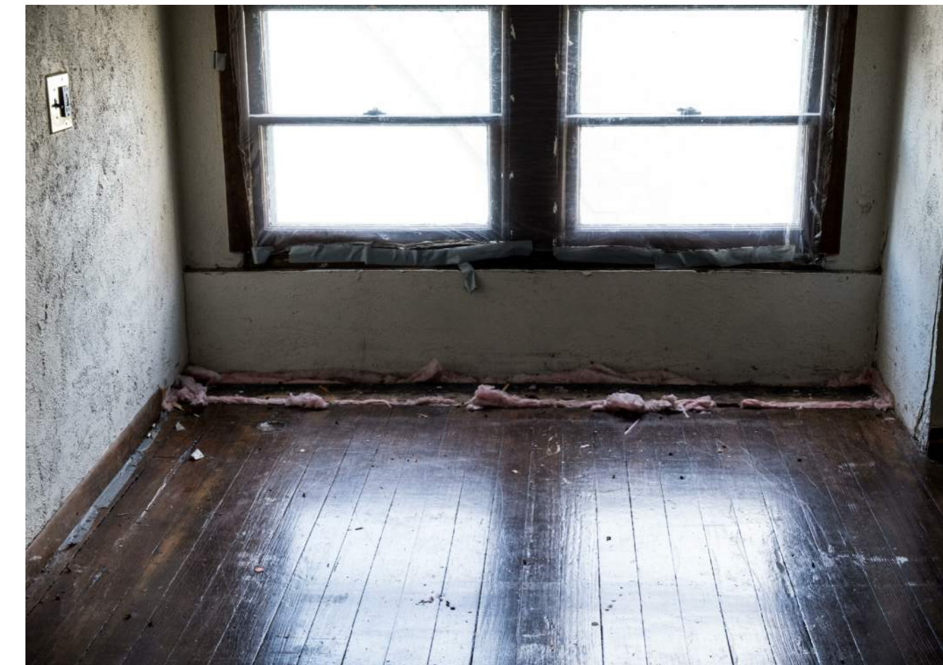
619 Lake Street - Interior No. 11
