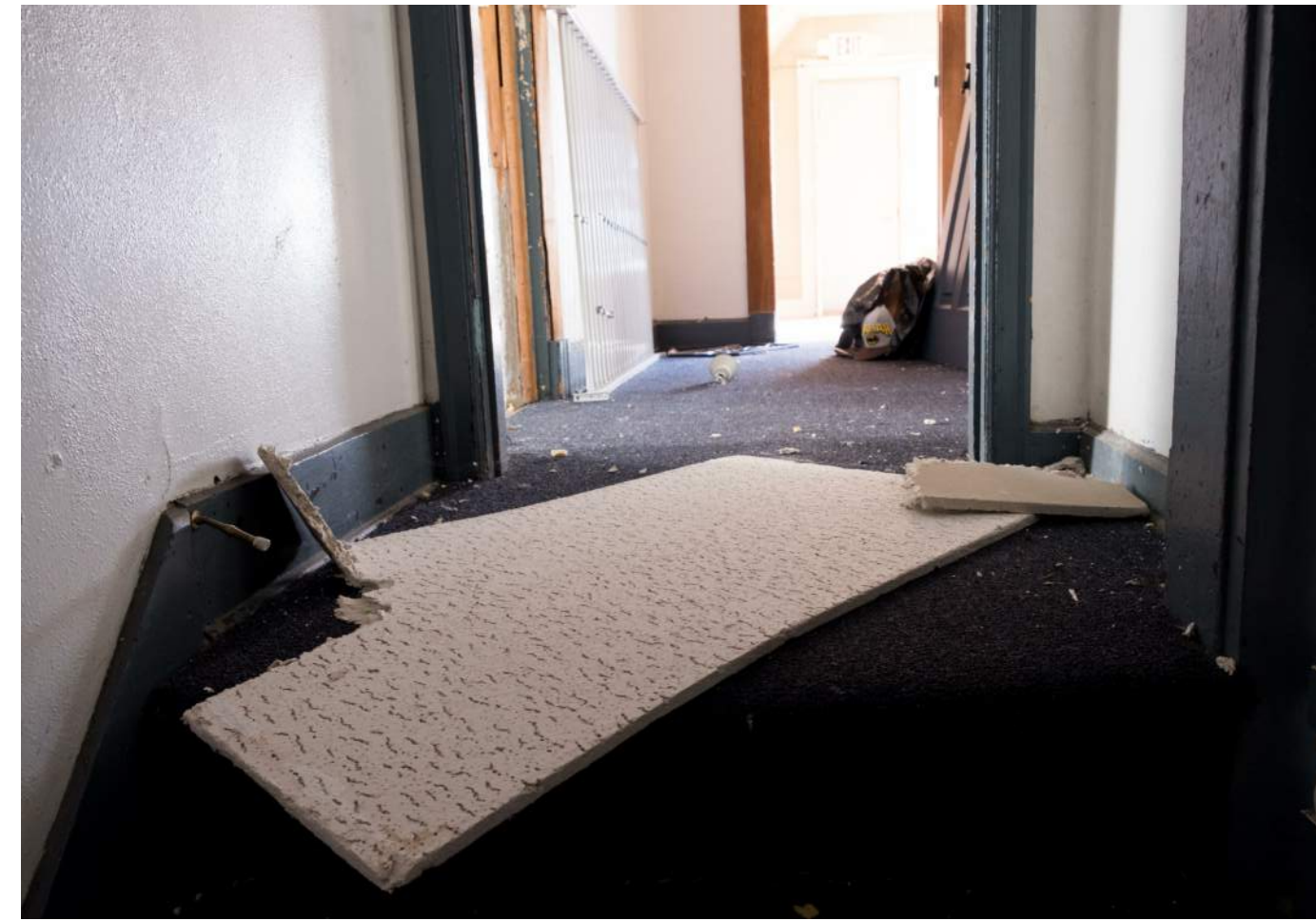
621 Lake Street - Interior No. 10
