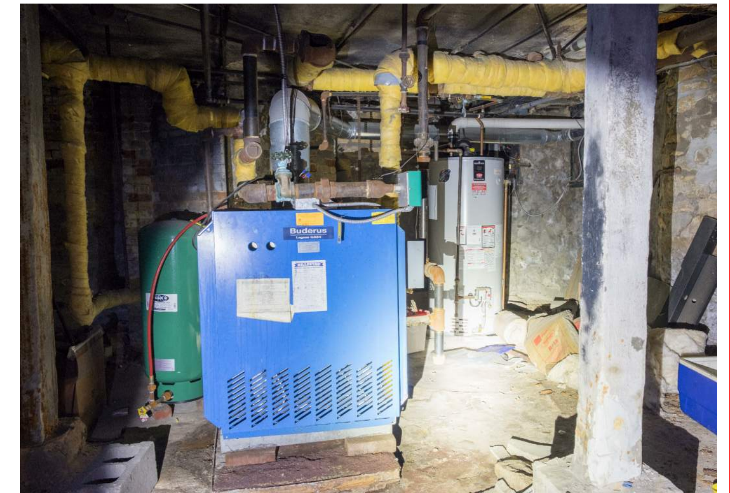
621 Lake Street - Interior No. 16
