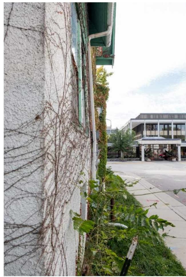
621 Lake Street - Exterior No. 9
