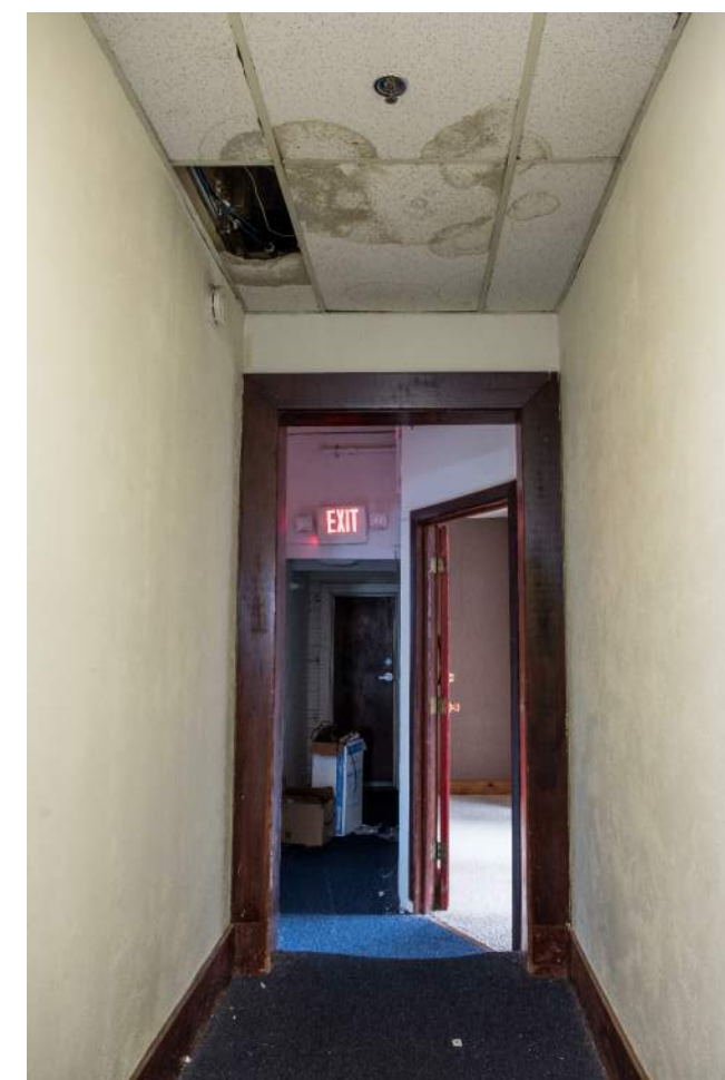
619 Lake Street - Interior No. 14
