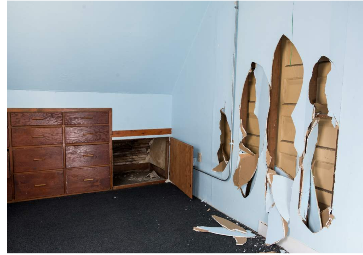
621 Lake Street - Interior No. 7
