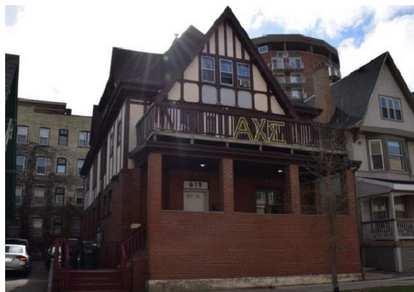
619 Lake Street - Exterior No. 2
