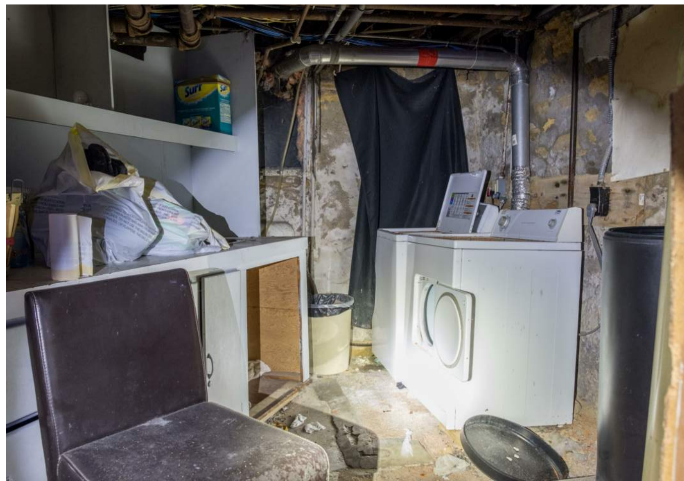
621 Lake Street - Interior No. 13
