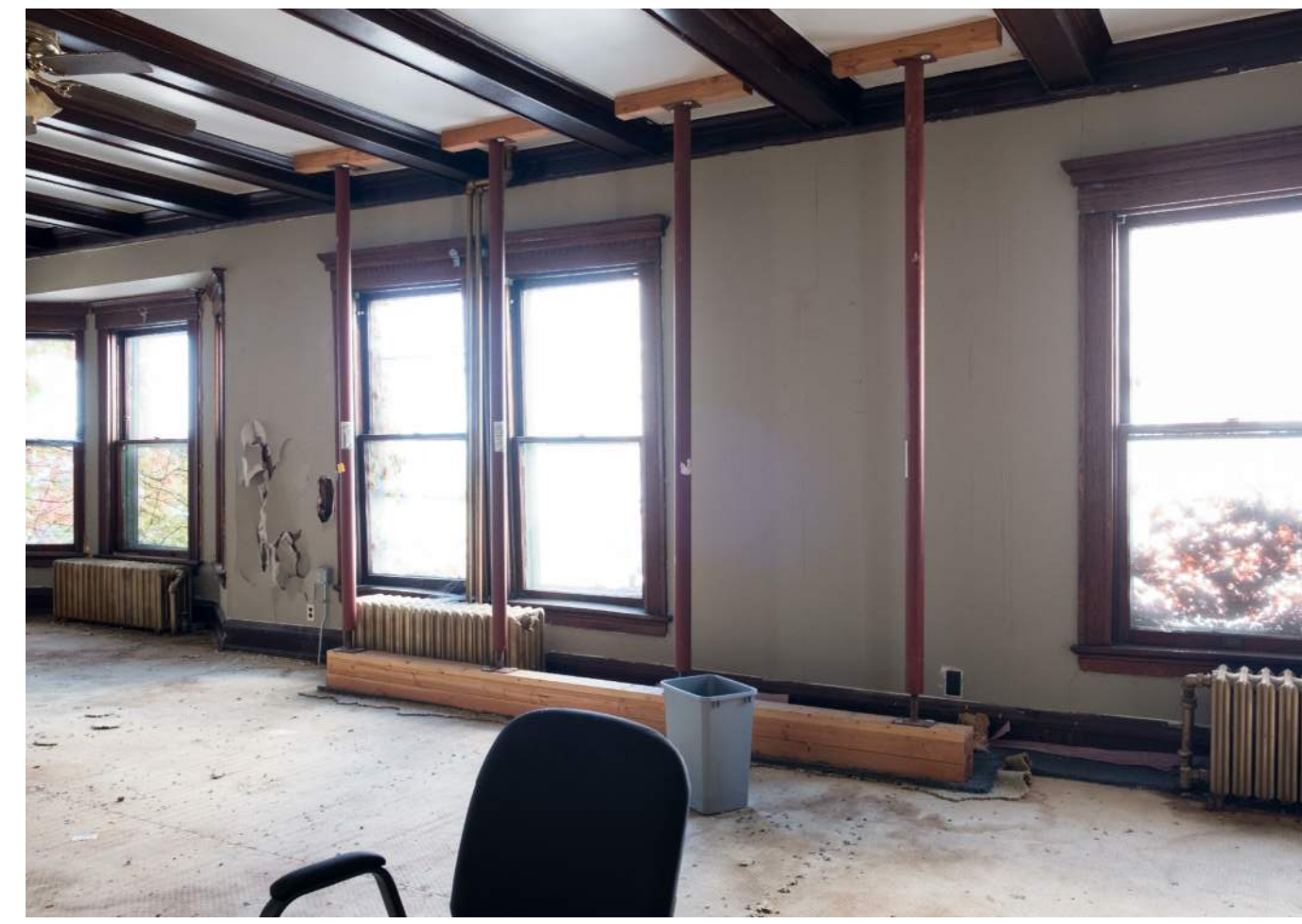
621 Lake Street - Interior No. 3
