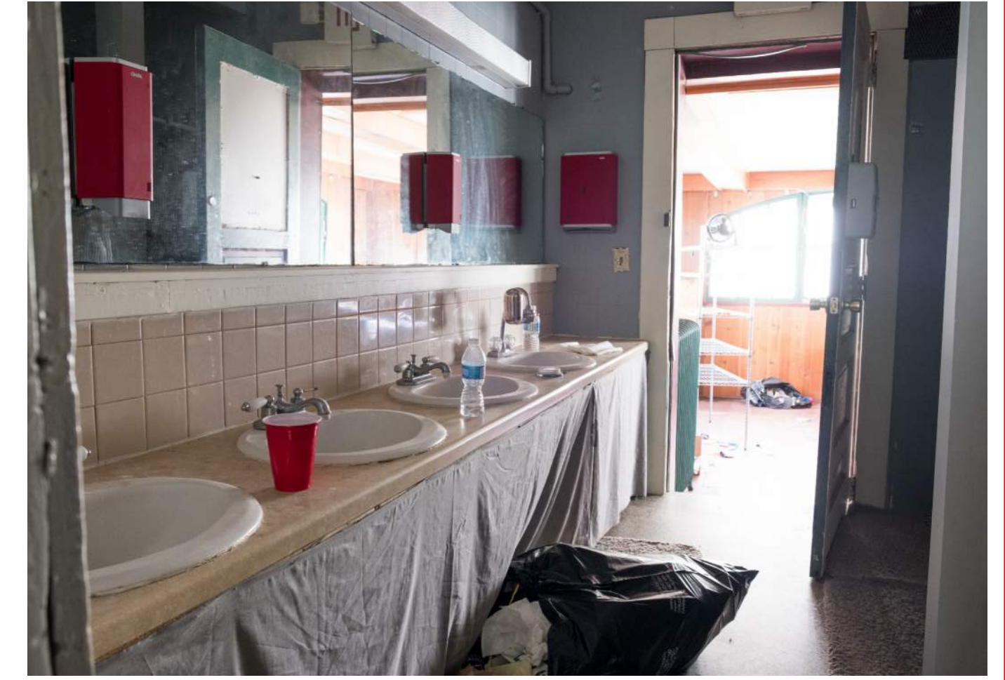
621 Lake Street - Interior No. 8
