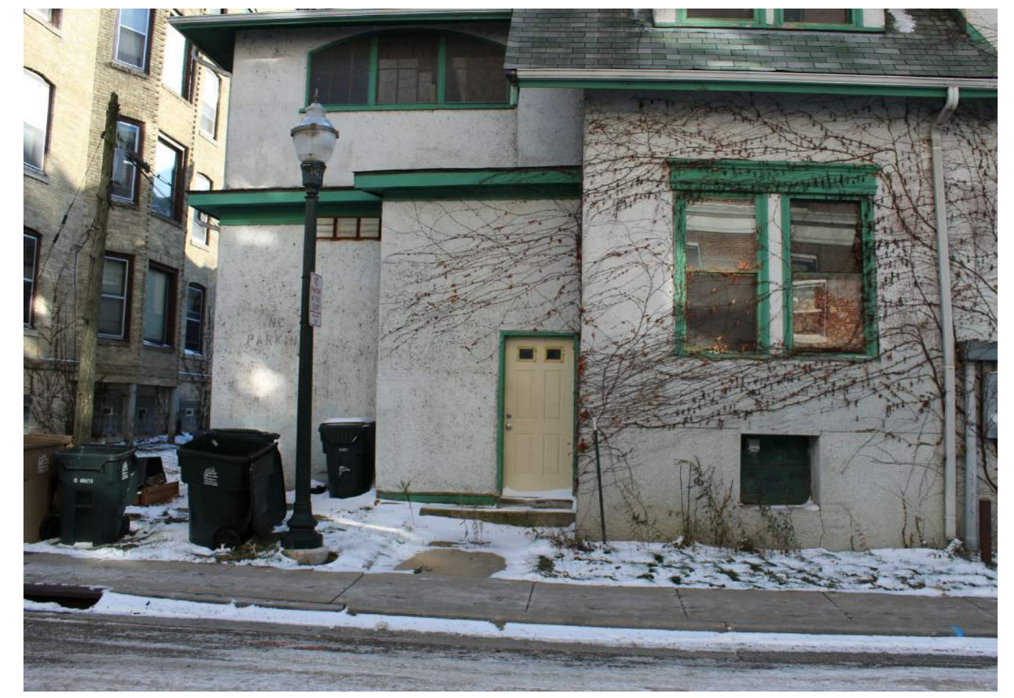
621 Lake Street - Exterior No. 4
