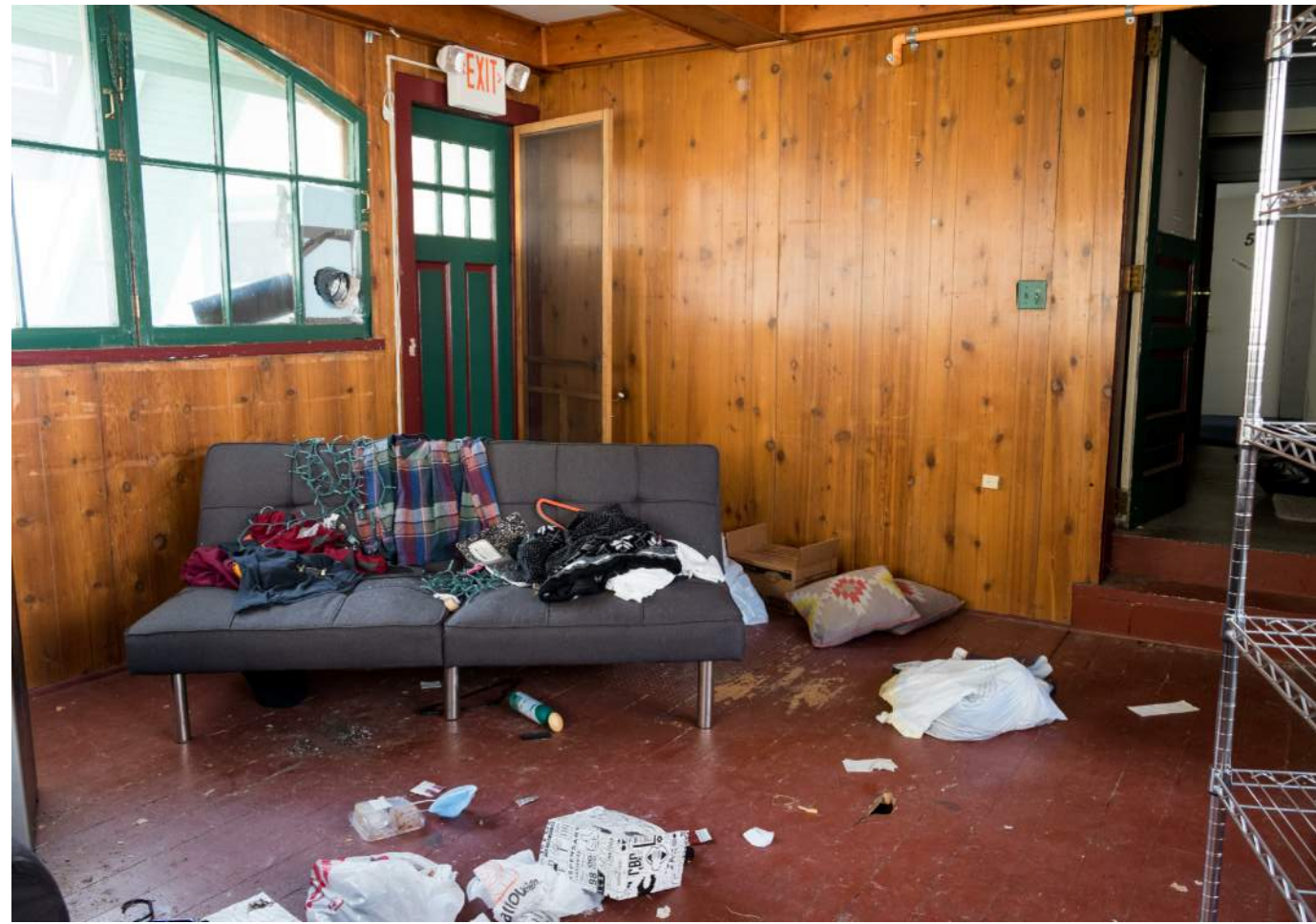
621 Lake Street - Interior No. 9
