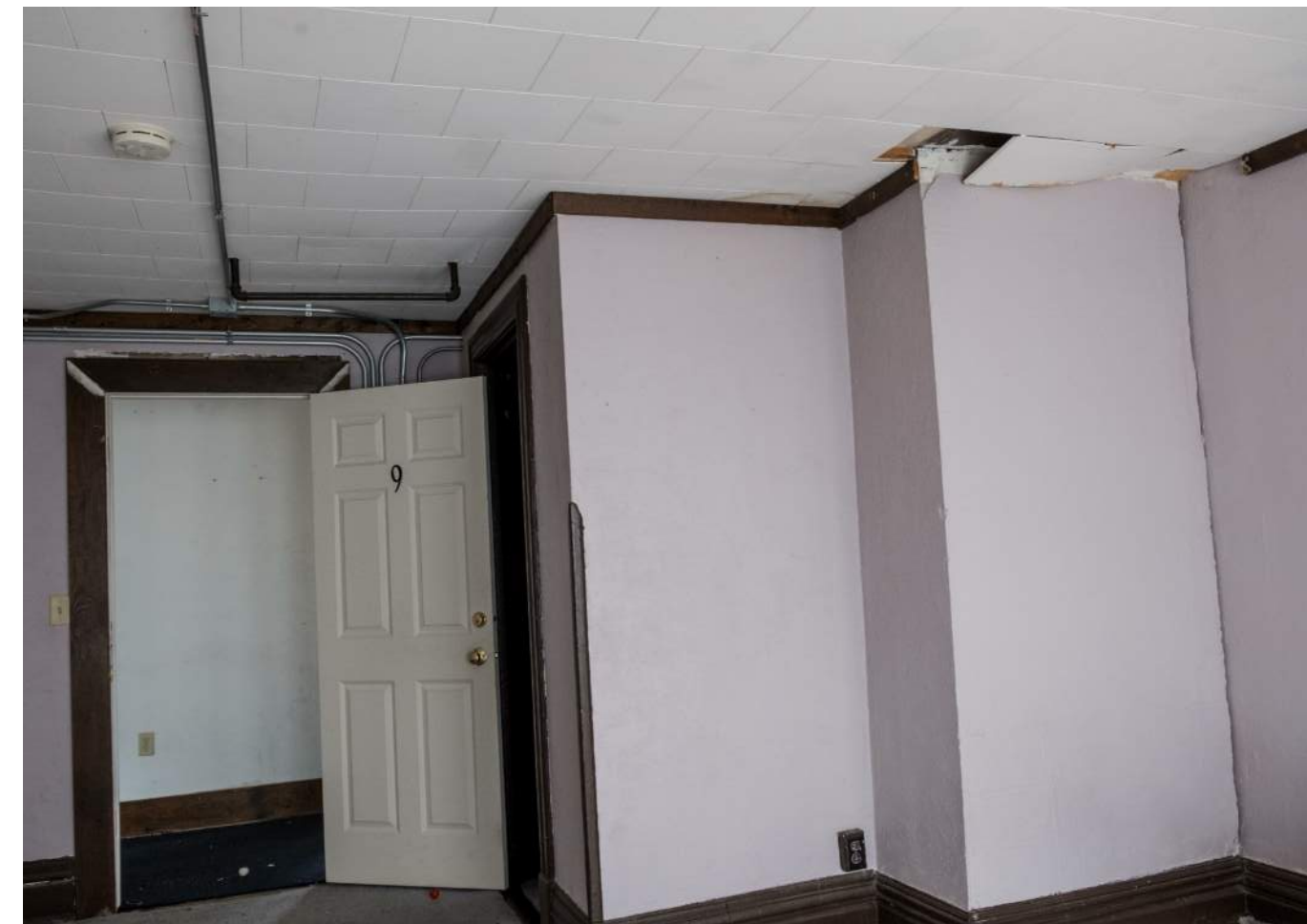
619 Lake Street - Interior No. 10
