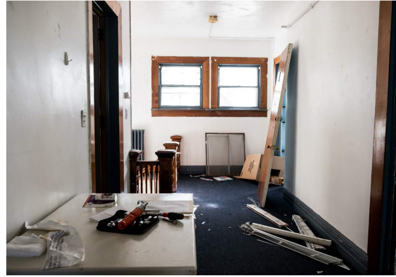
621 Lake Street - Interior No. 6
