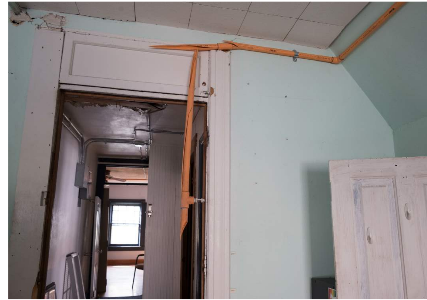
621 Lake Street - Interior No. 11
