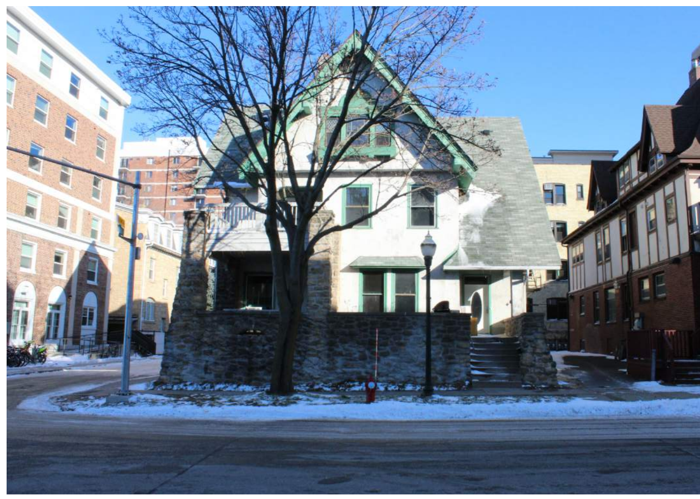
621 Lake Street - Exterior No. 1
