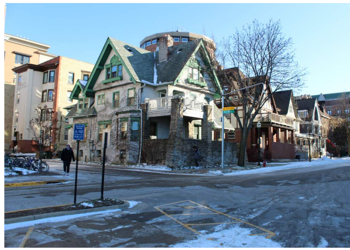
621 Lake Street - Exterior No. 2
