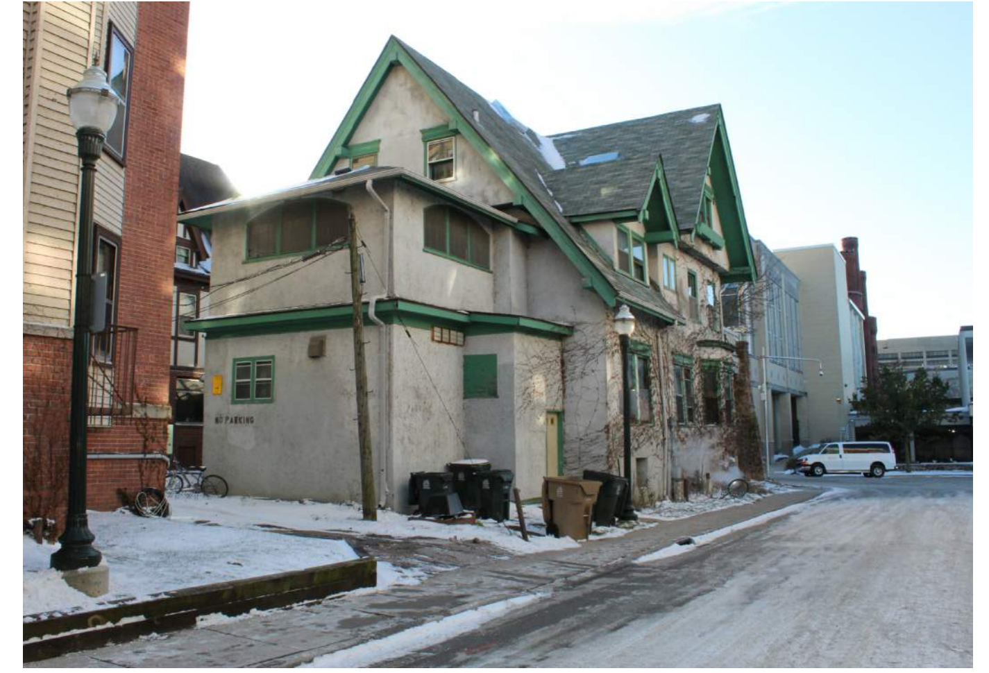
621 Lake Street - Exterior No. 8
