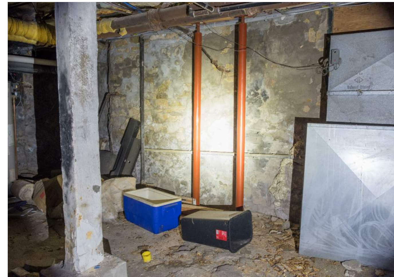
621 Lake Street - Interior No. 15
