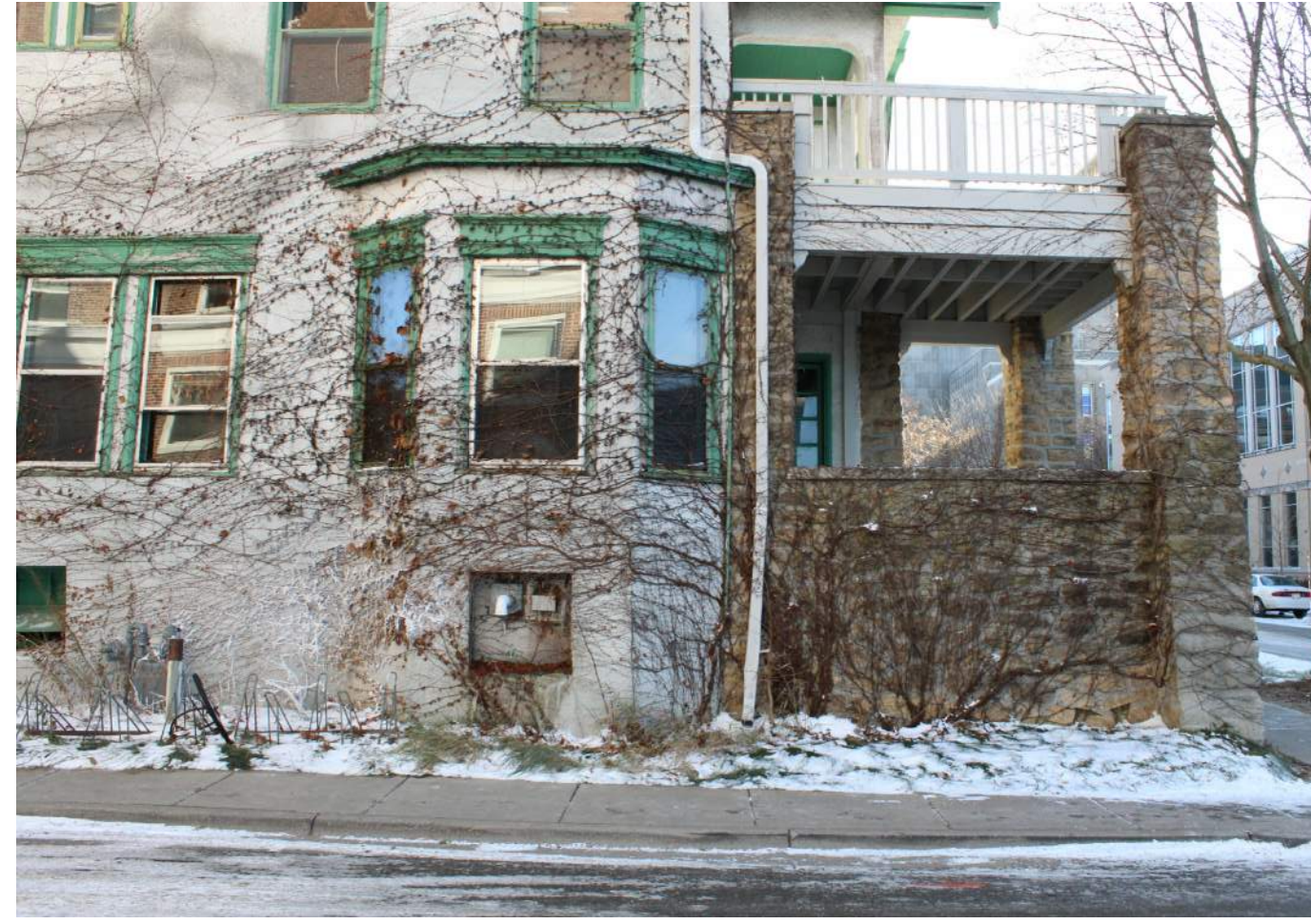
621 Lake Street - Exterior No. 6
