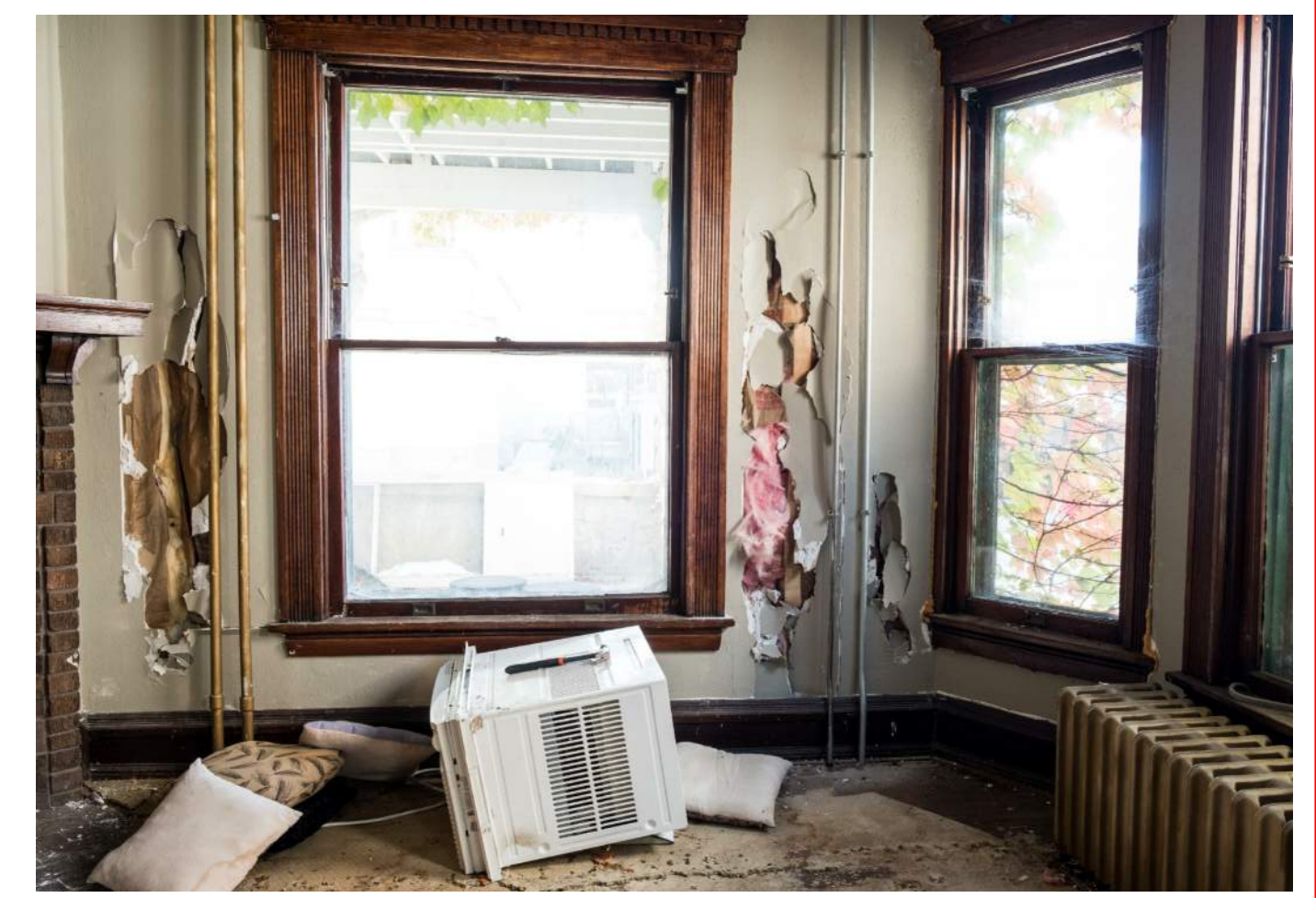
621 Lake Street- Interior No. 4
