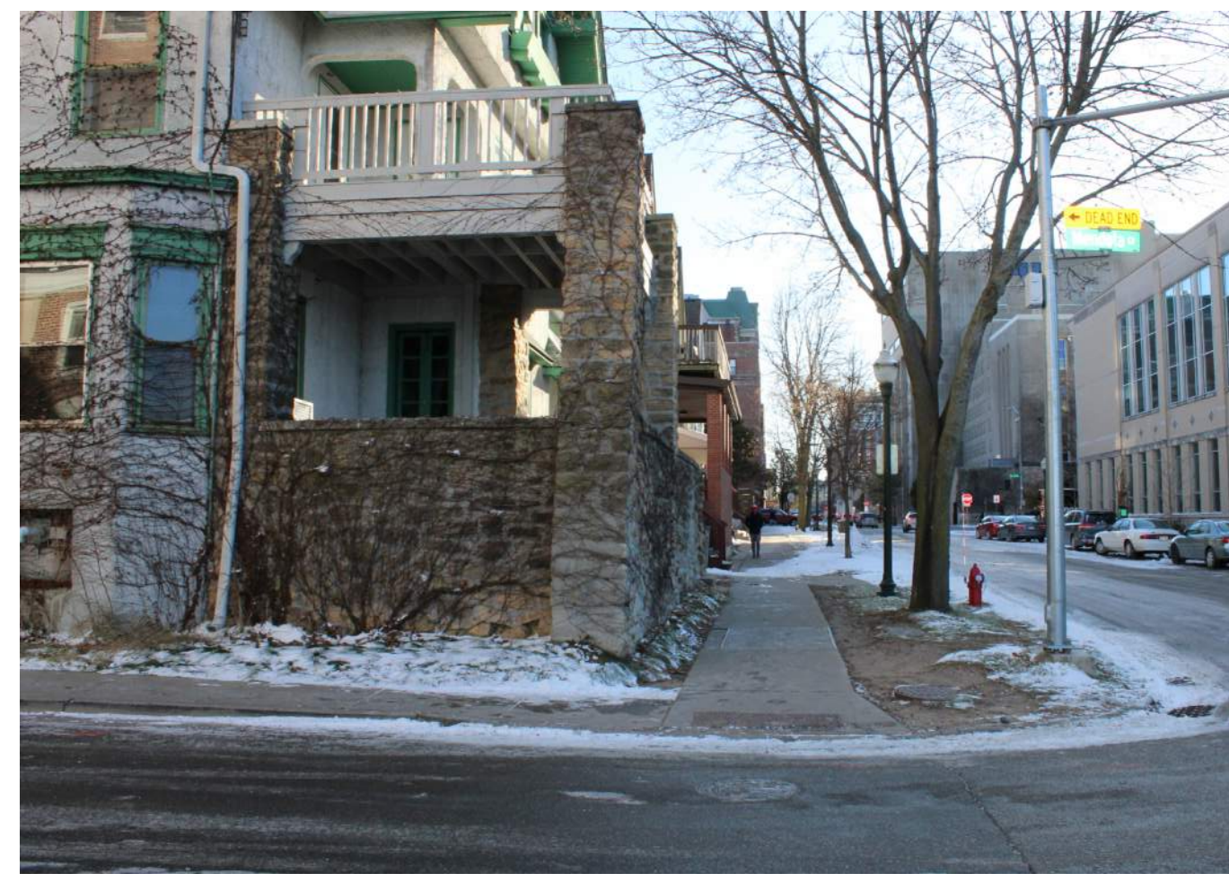
621 Lake Street - Exterior No. 3
