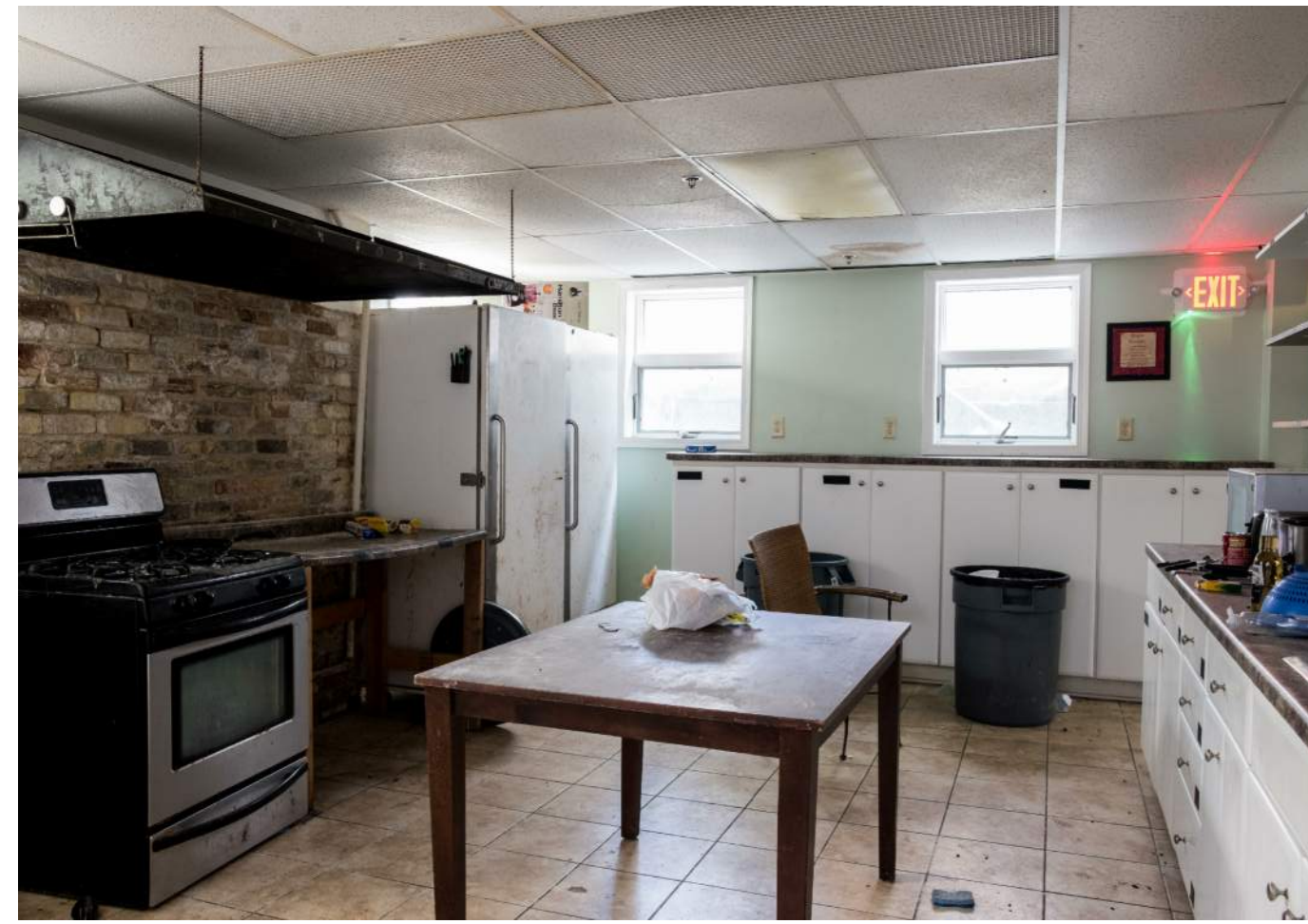
619 Lake Street - Interior No. 1
