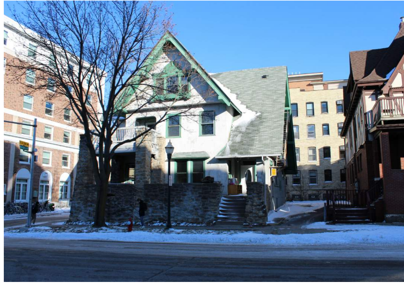
621 Lake Street - Exterior No. 5
