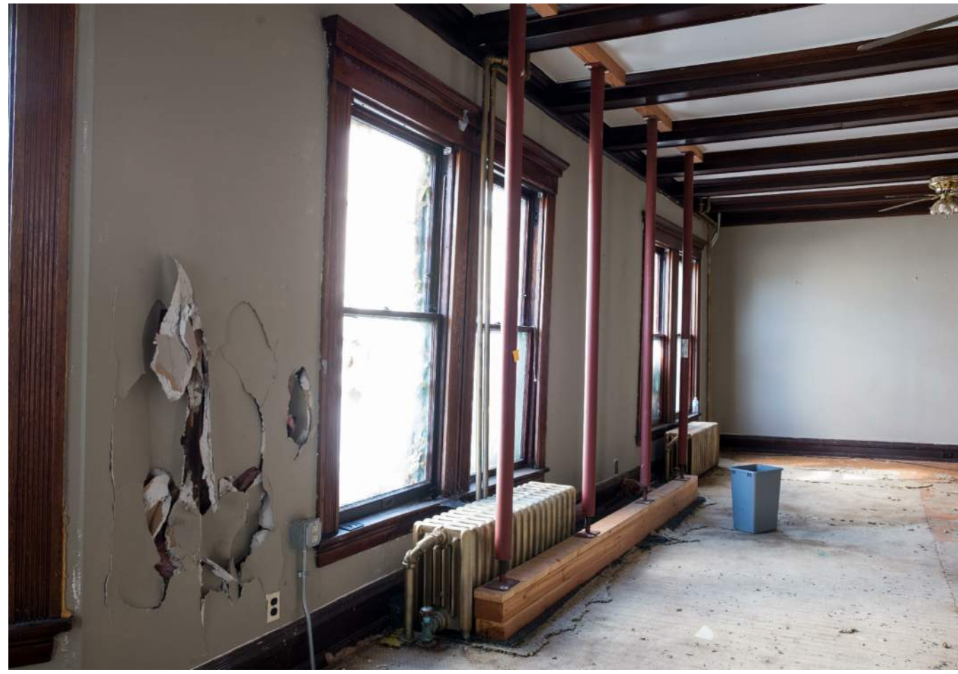
621 Lake Street - Interior No. 5
