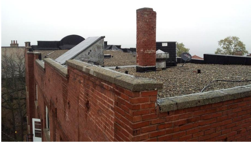
Image 1.59 The roof is a low-slope design consisting of a stone-ballasted EPDM (rubber) membrane bordered with continuous brick masonry parapets with precast concrete caps.
