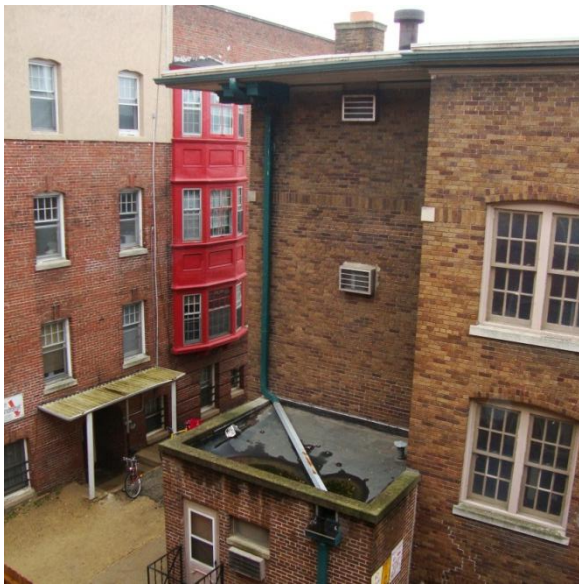
Image 1.24 View of the east side of 625 Henry Street (right) and the north side of 621 Henry Street (left).
