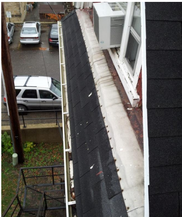
Image 1.9 Gutters and downspouts consist of prefinished sheet metal; they are sound. They appear newer and could possibly be reclaimed
