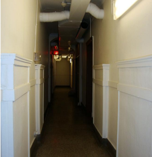
Image 1.62 View of a typical corridor.
