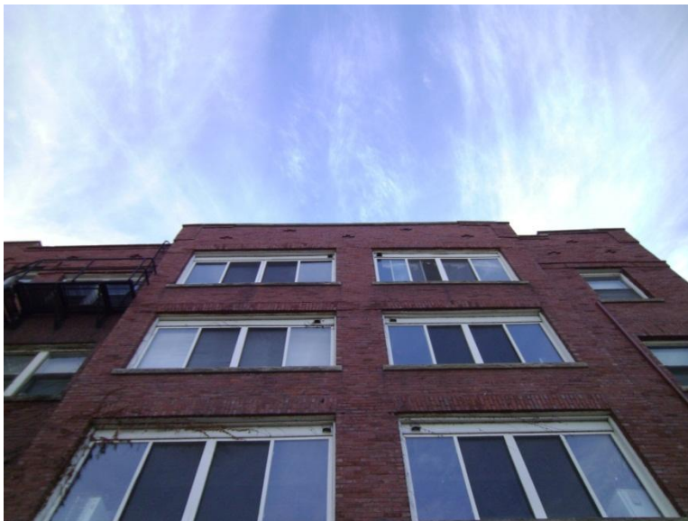
Image 1.67 View of the east façade of 145 Iota Court
