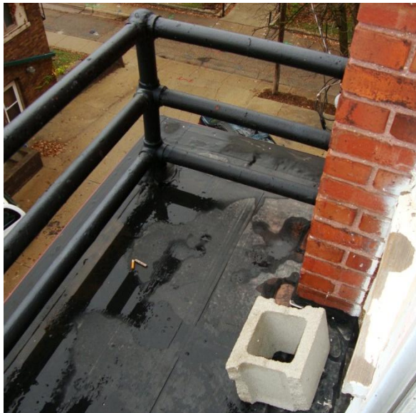
Image 1.56 West facing balcony deck.
