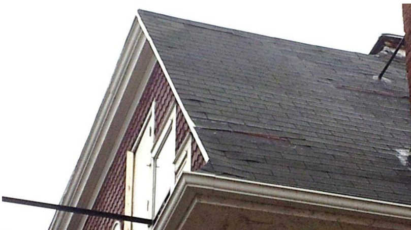
Image 1.7 The roof is a gable design with complementary gabled dormers. The roofing systems include roll membrane (asphaltic), (asphaltic) shingle, and metal.
