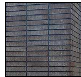
3) CONCRETE: BRICK TEXTURE, STAINED CHARCOAL
