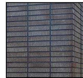
3) CONCRETE: BRICK TEXTURE, STAINED CHARCOAL
