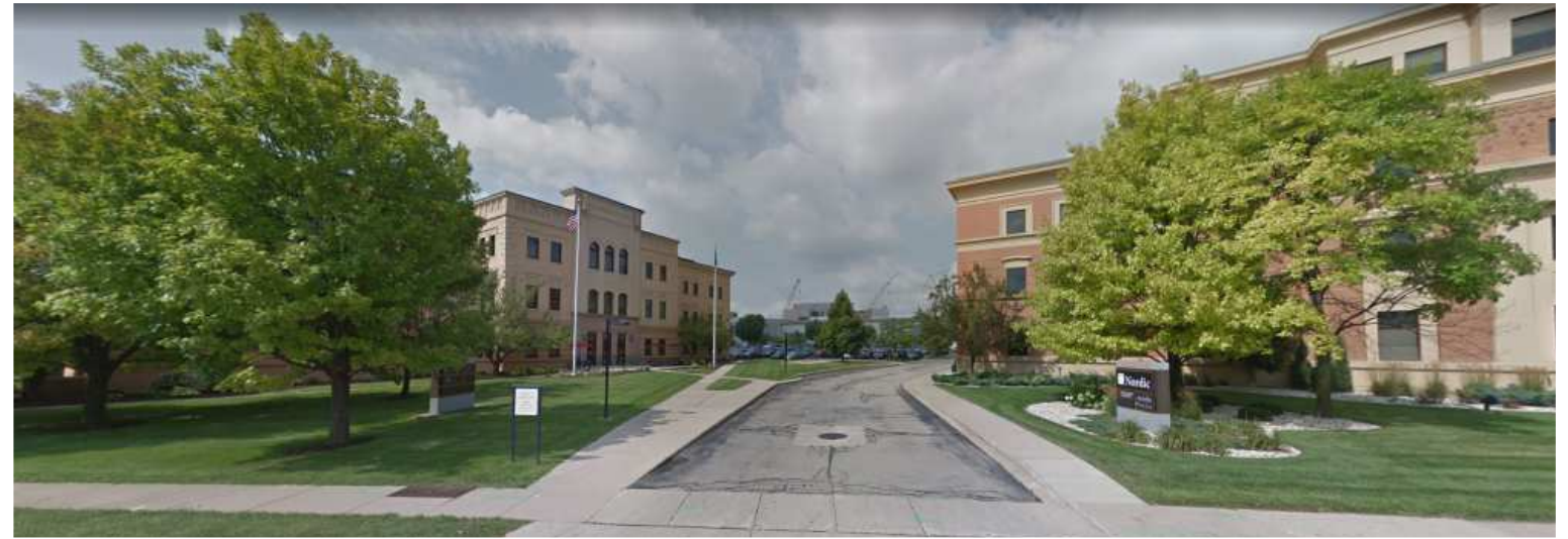
VIEW NORTH FROM REGENT STREET
