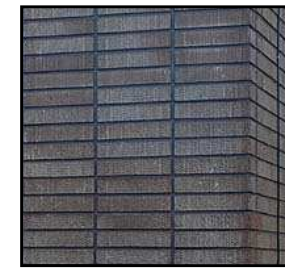
3) CONCRETE: BRICK TEXTURE, STAINED CHARCOAL
