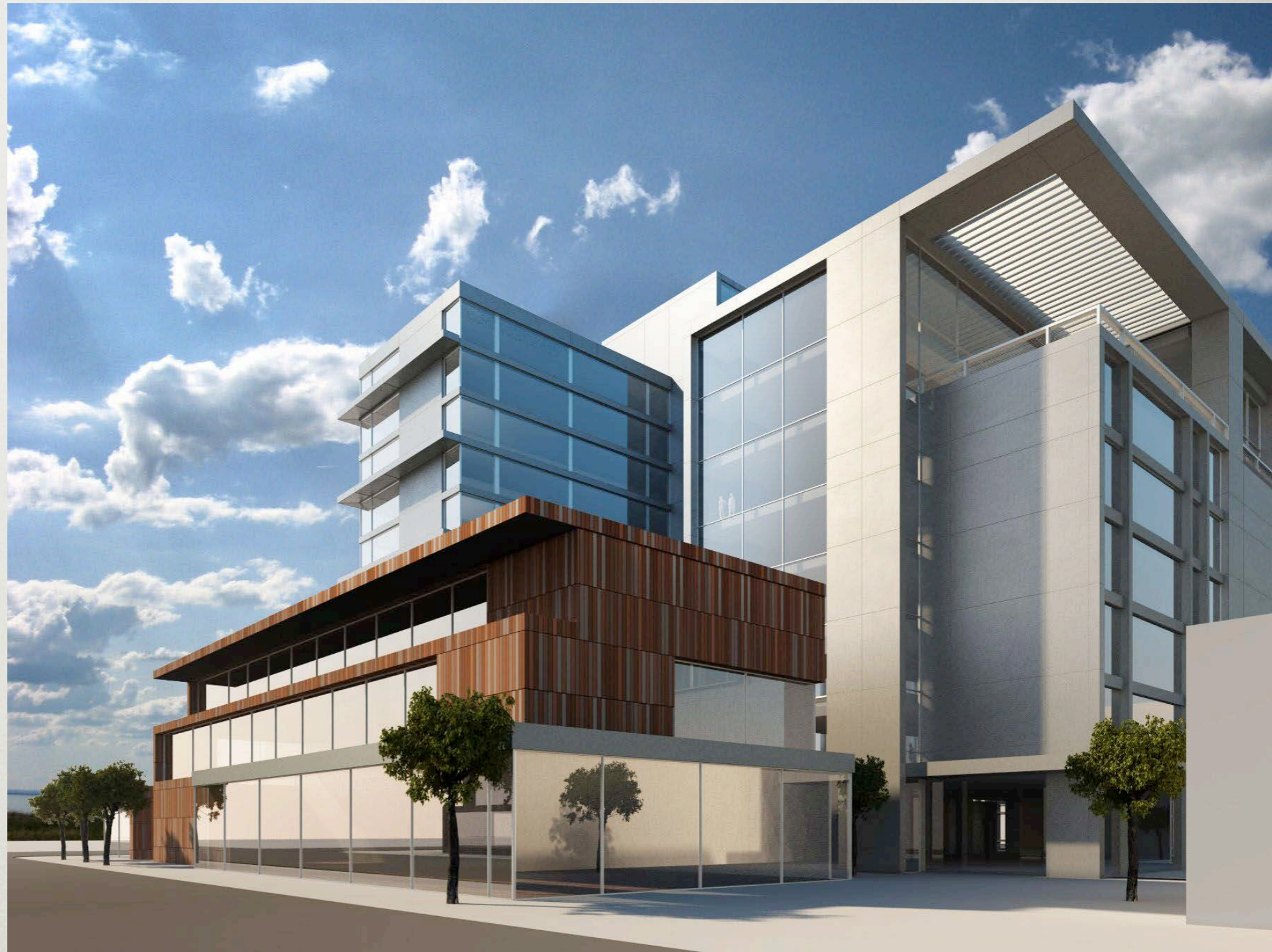
view from east main
