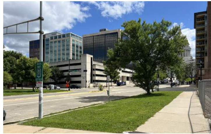
Wisconsin/Dayton Parking Garage
