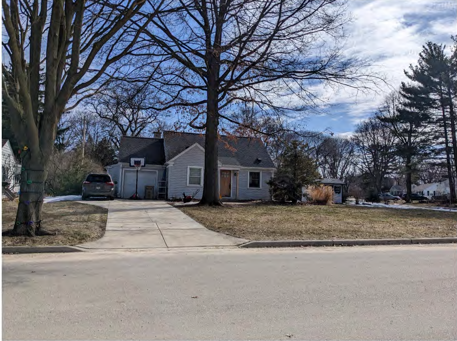
Front West Elevation – View from Westmorland
