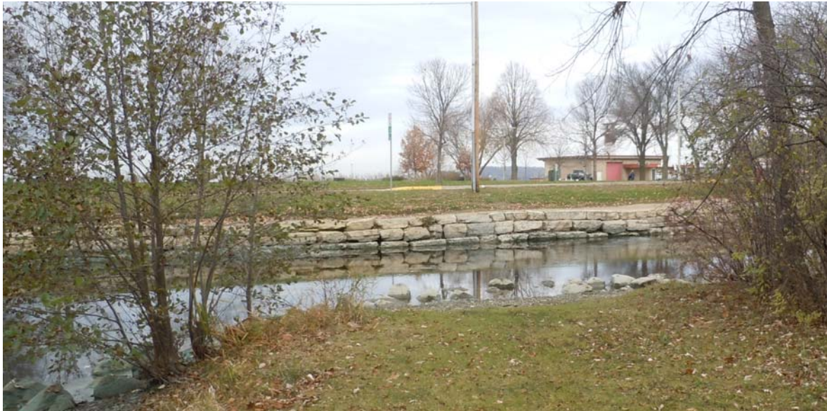
Figure 3: Existing, cut, limestone steps. The proposed steps will be similar in appearance to these. However, since the shoreline where they'll be placed is shorter than this area, only two rows of blocks will be used.
