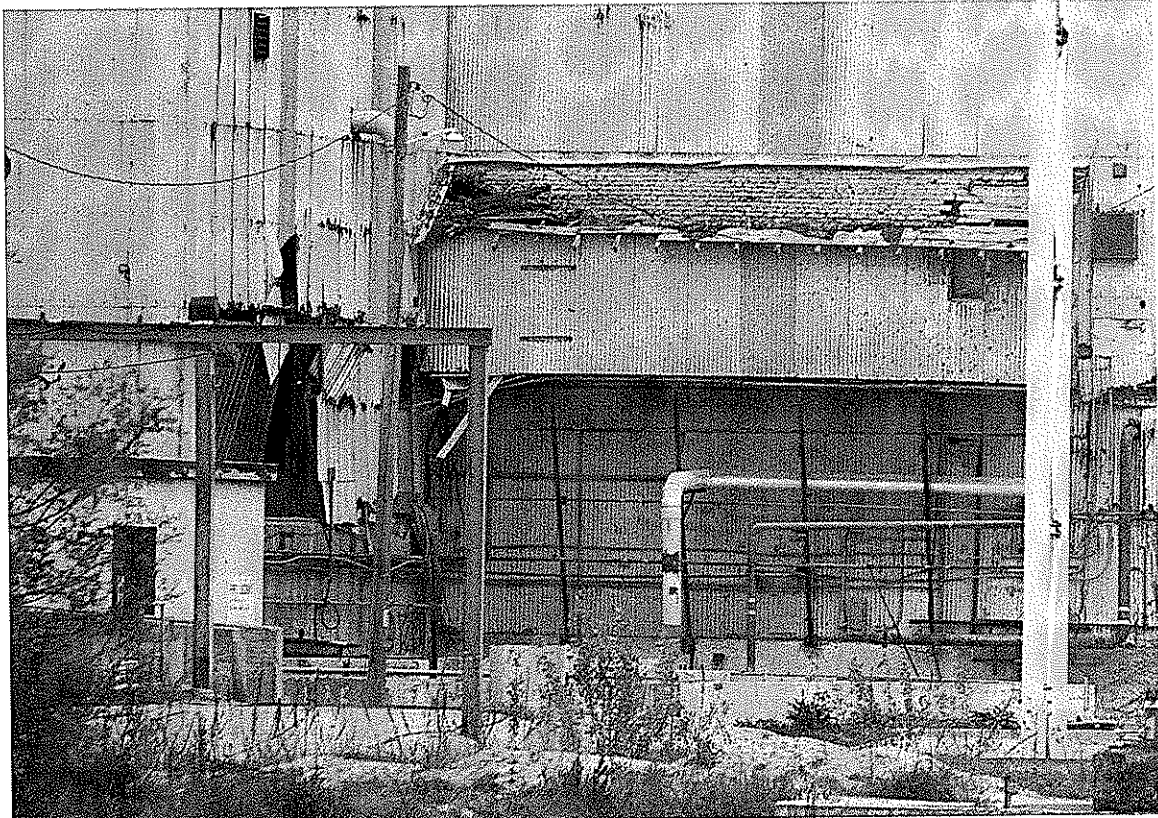
Condition of walls and doors on exterior of granulation building, May 2008
