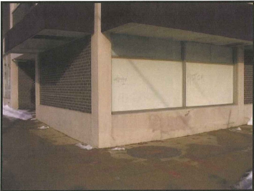
Street level facade
