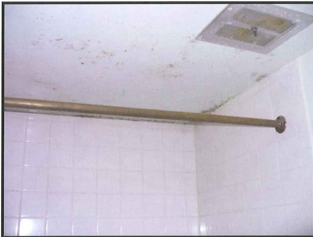
Typical apartment bathroom ceiling
