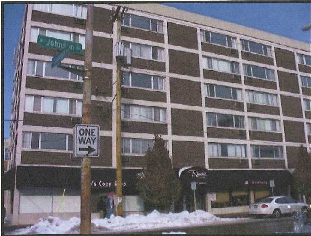
Front exterior along Johnson
