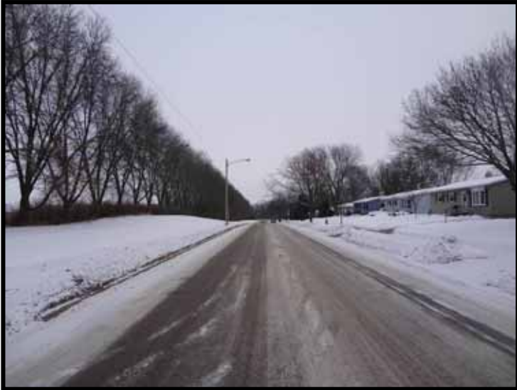
Looking East along Tennyson Lane
