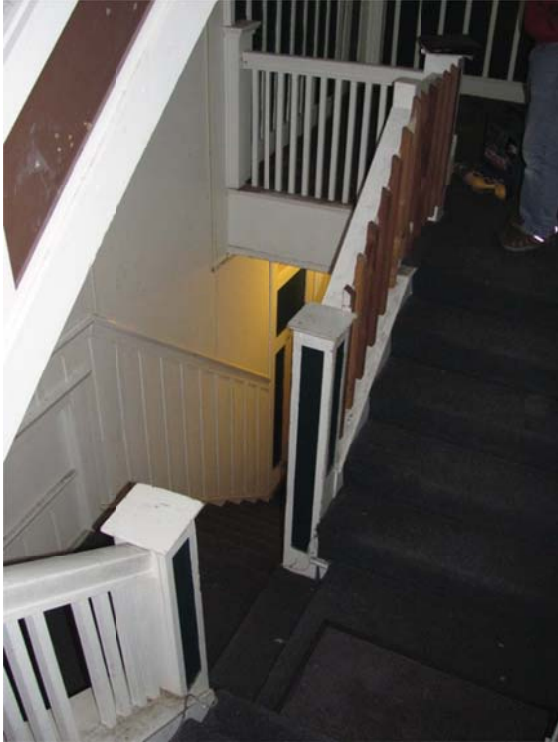
Figure 19. The central part of the interior at the second and third floors contains a complex switch-back staircase.
