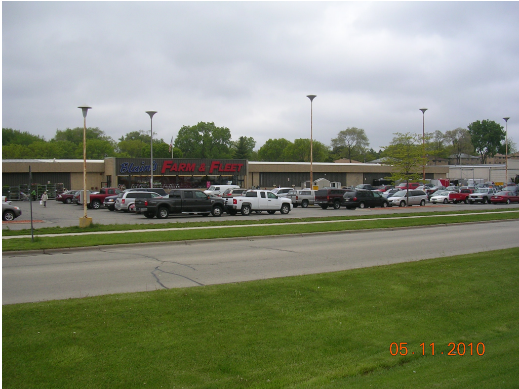
Mid Portion of East Elevation
