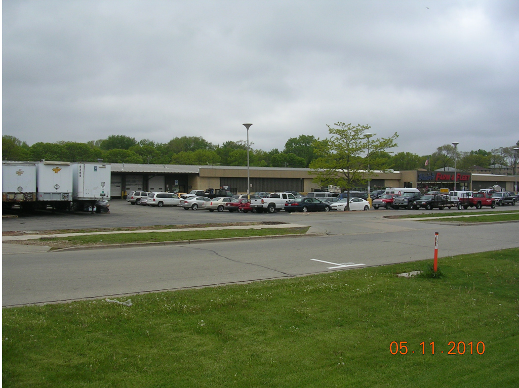
South Portion of East Elevation
