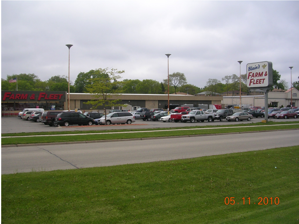
North Portion of East Elevation Including Existing Road Sign
