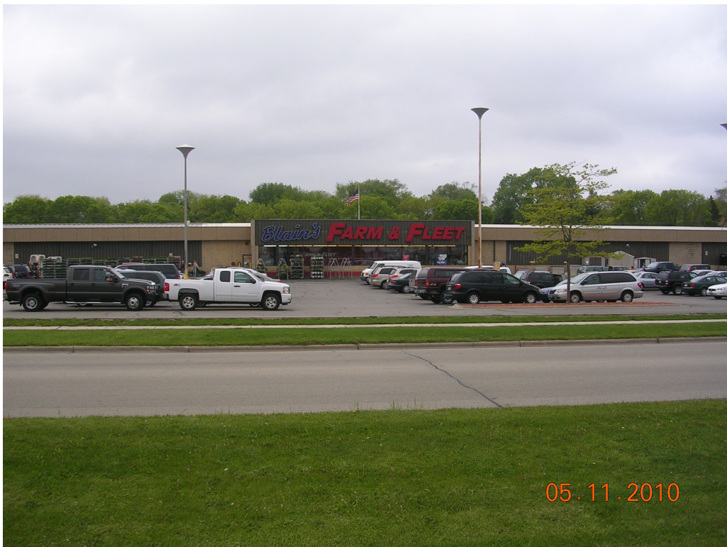
Vestibule (Straight one) East Elevation
