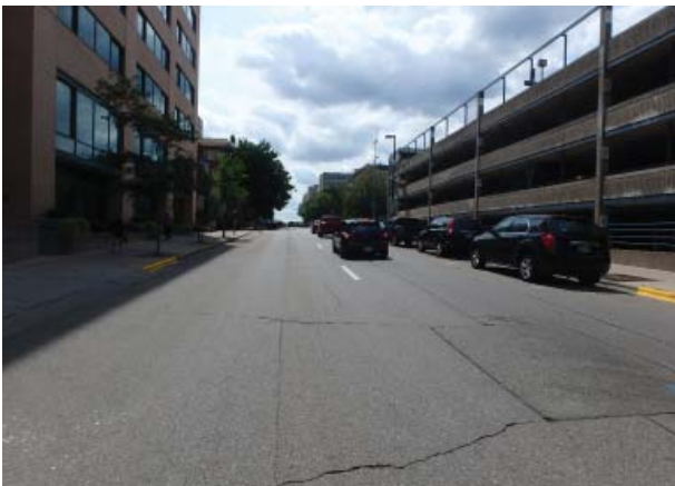
West Wilson Street (Good to Fair condition)
