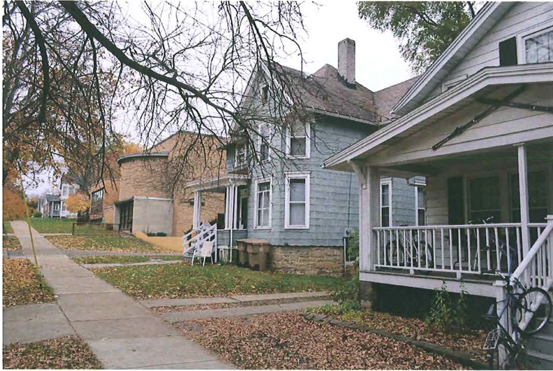
Image 4 - Site from sidewalk along Randall Street looking South
