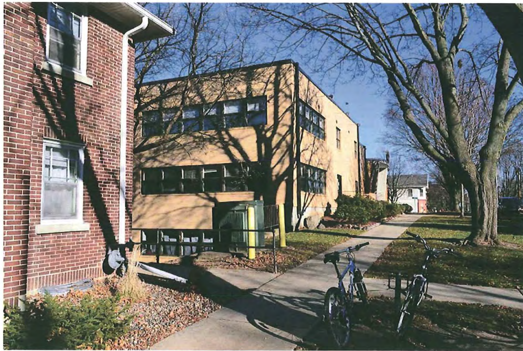
Image 2 - Along sidewalk at Mound Street looking East
