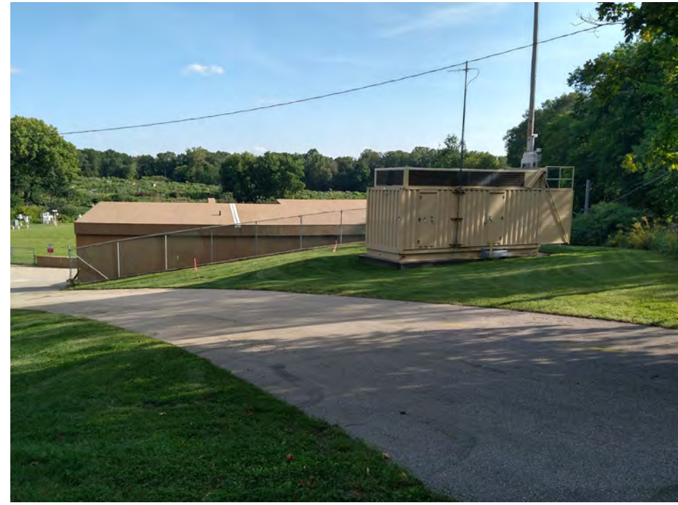
Site viewed from existing driveway, looking southeast
