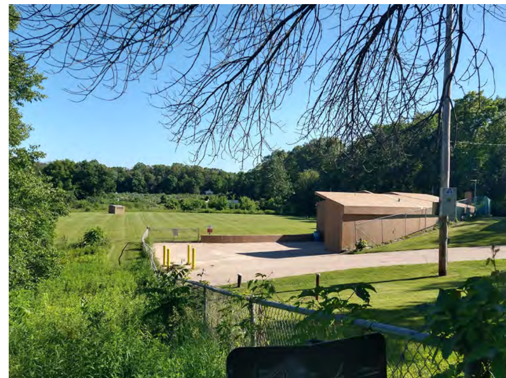
View of existing building from Lakeshore Preserve Trail, looking southwest
