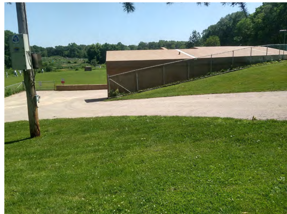
Existing driveway and building, looking south
