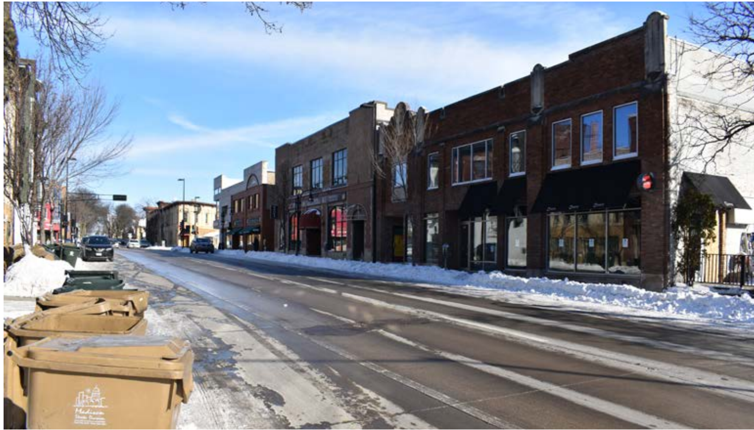
GORHAM STREET LOOKING NORTHEAST TOWARD PROJECT SITE
