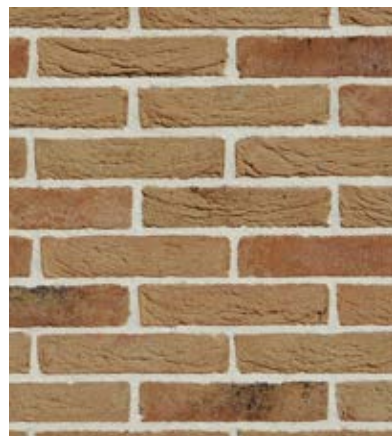
EXISTING FACADE BRICK
