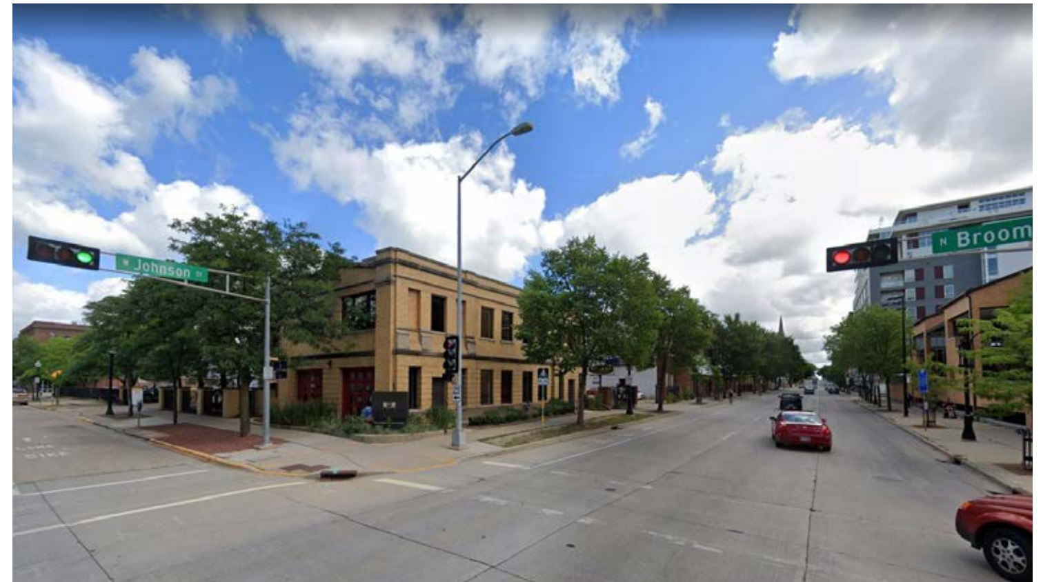
CORNER OF JOHNSON STREET AND BROOM STREET LOOKING NORTH TOWARD PROJECT SITE
