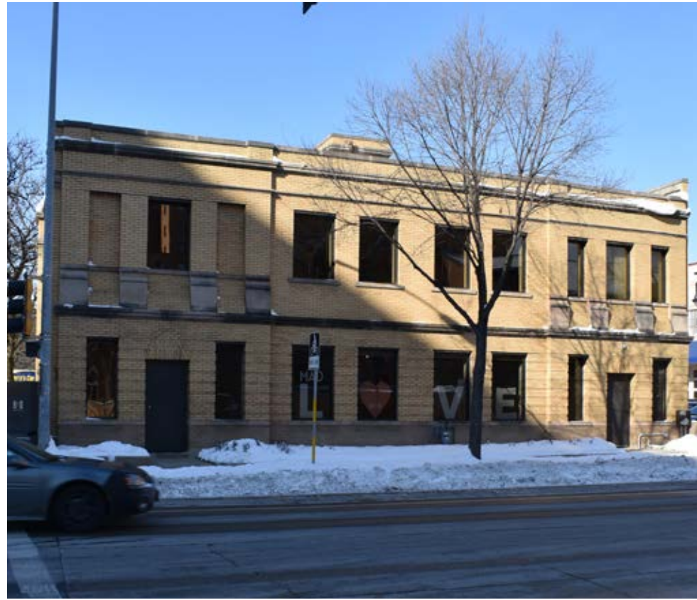
301 W JOHNSON STREET
