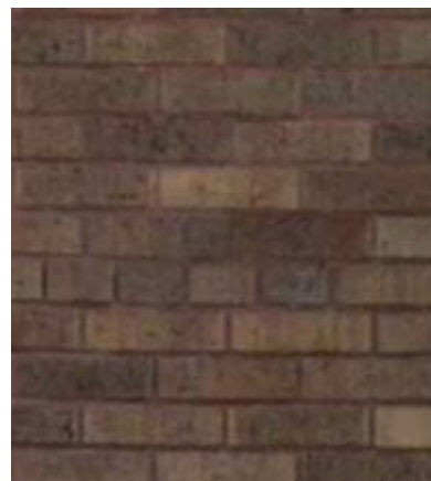
EXISTING FACADE BRICK
