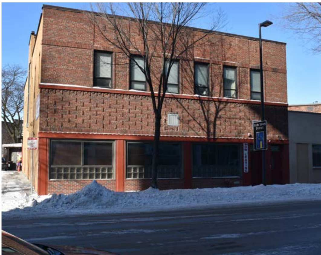
303 STATE STREET (W JOHNSON ST FACADE)
