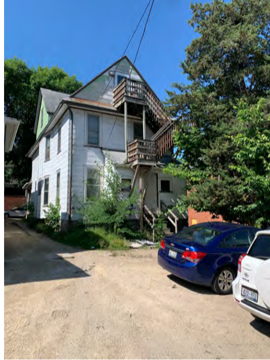
View from Rear yard
