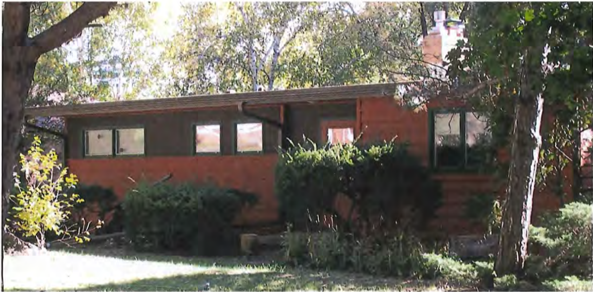
5013 Tomahawk Trail. A flat roof and effective use of a color and material transition that complements the simple architecture.
