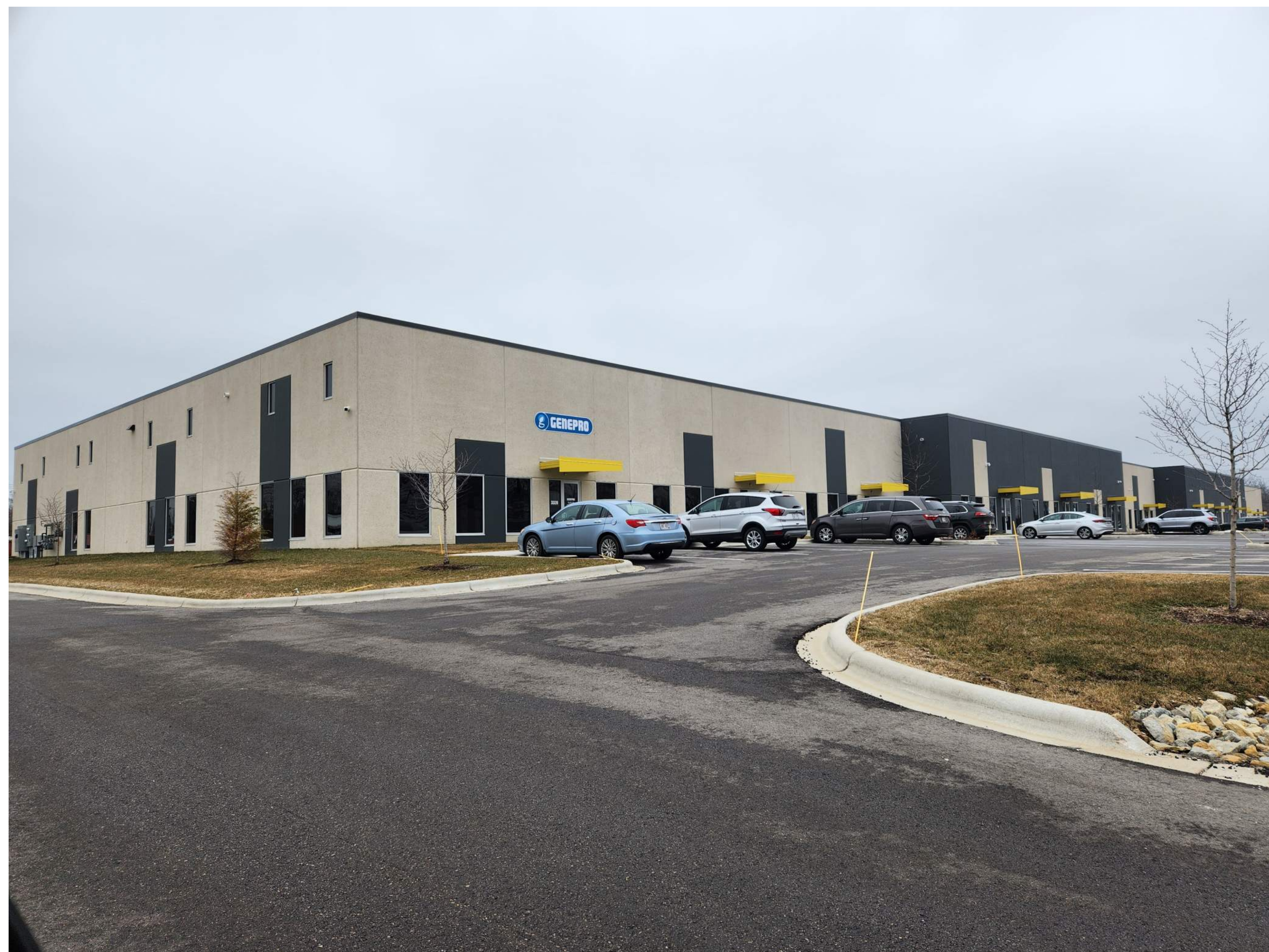
WAREHOUSE ACROSS DAIRY DRIVE
