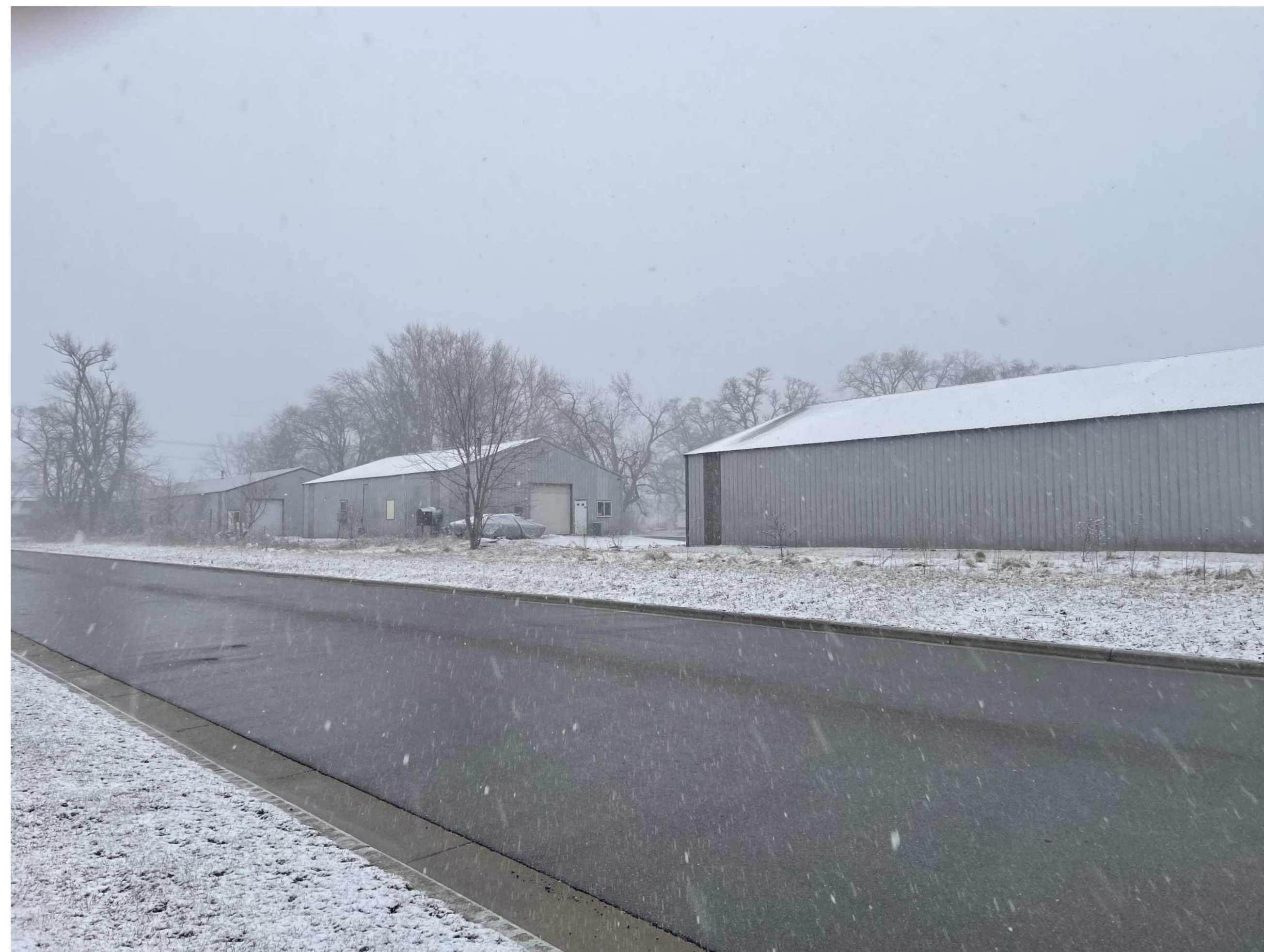
METAL BUILDINGS TO THE NORTH OF 3351 DAIRY DRIVE
