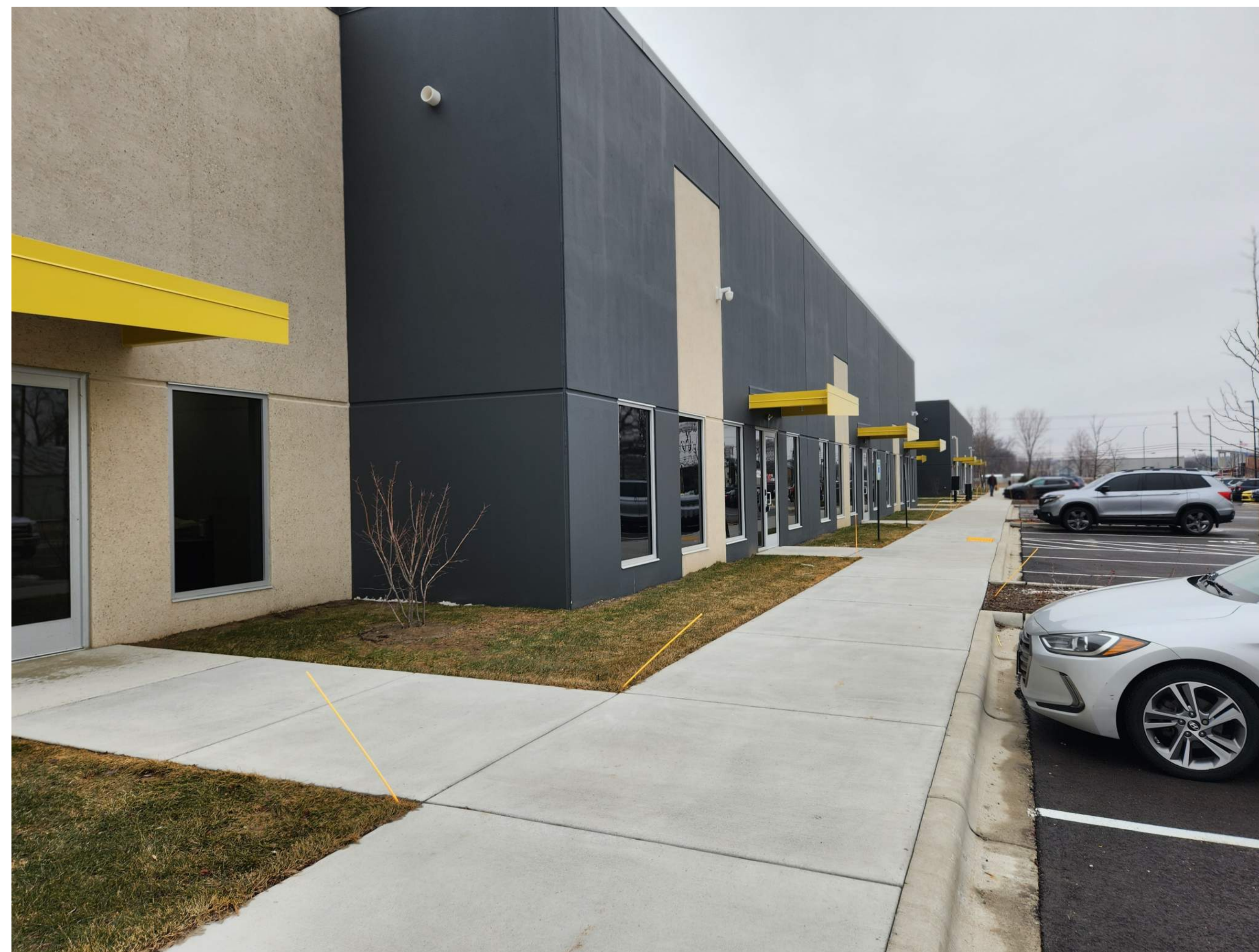
WAREHOUSE ACROSS DAIRY DRIVE DETAIL
