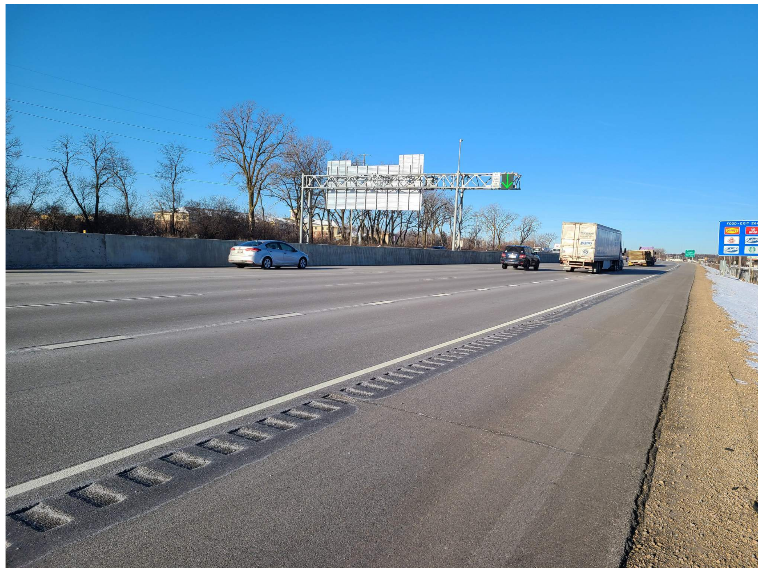
CONCRETE MEDIAN BLOCKS VIEW FROM EASTBOUND BELTLINE
