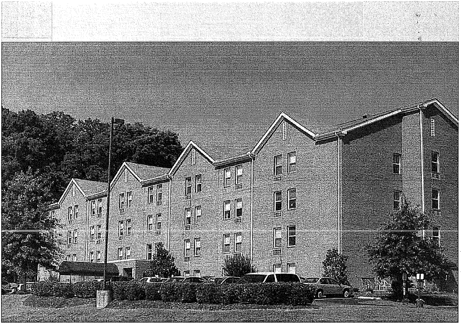
Heartland Christian Tower, Nashville, TN (Photo Credit: Staci Bergeron)
