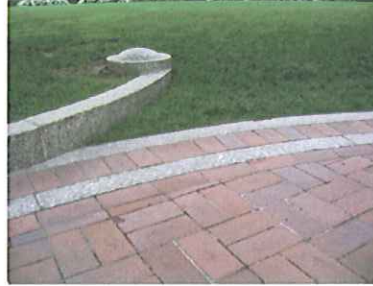
4 Lawn with Granite Curb and Brick Paving with Granite Trim Details SCALE: 1/2"
