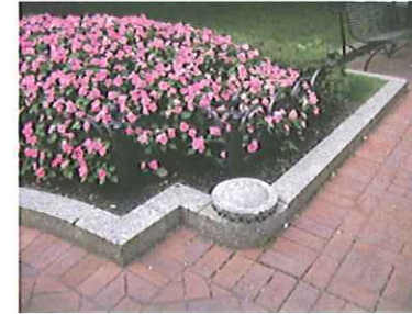
3 Planted Area with Granite Curb Detail SCALE: 1/2"
