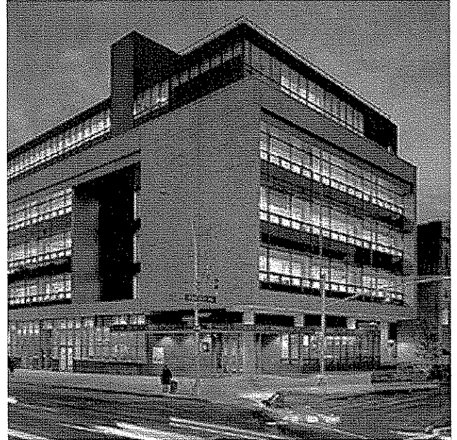
A combination of durable materials creates a contemporary expression that also conveys permanence
