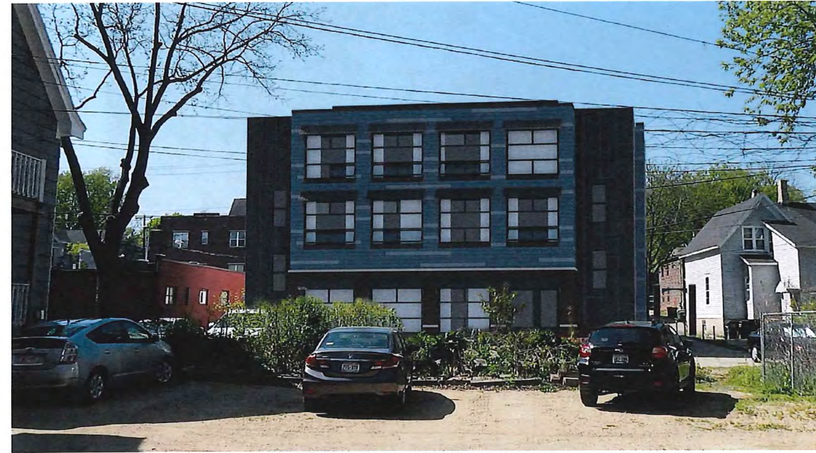
VIEW LOOKING NORTH-EAST FROM BACK LOT
