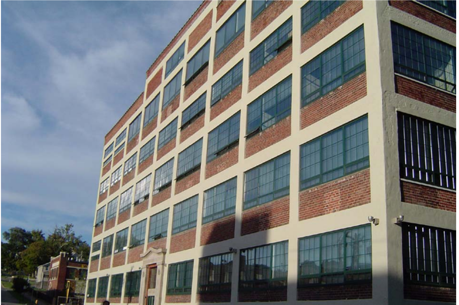
Alexander Company Project Profile: Davenport Lofts
