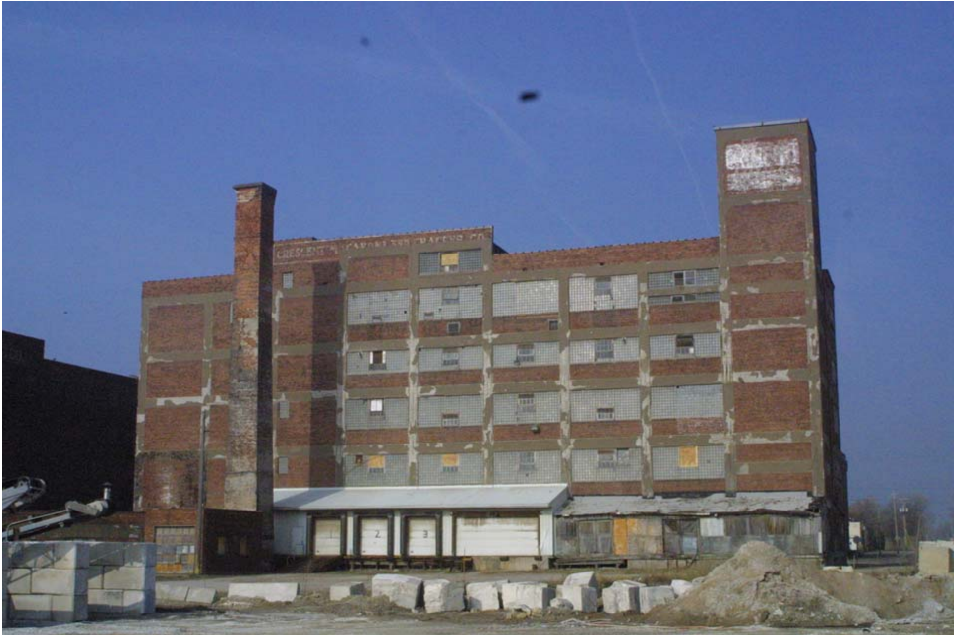
Alexander Company Project Profile: Davenport Lofts
