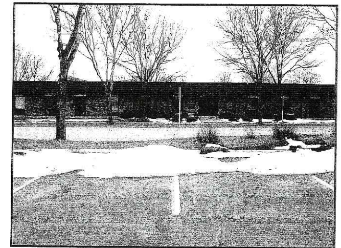
CENTRAL OUTLOT SITE LOOKING SOUTH
