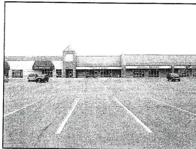
CENTRAL OUTLOT SITE LOOKING NORTH
