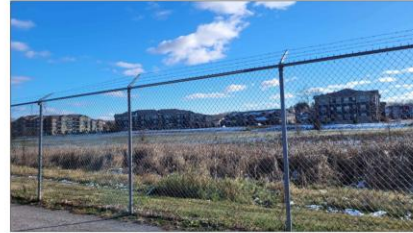
8' GALVANIZED CHAINLINK W/ BARBWIRE (C)
