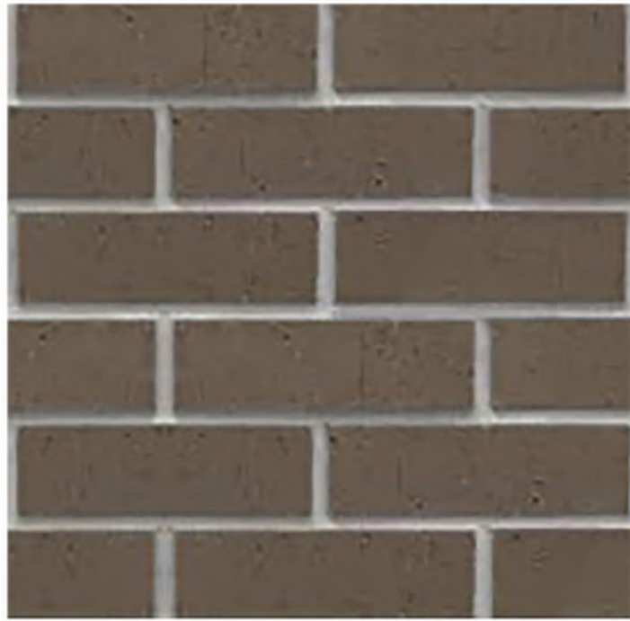
MASONRY VENEER - RUNNING BOND
