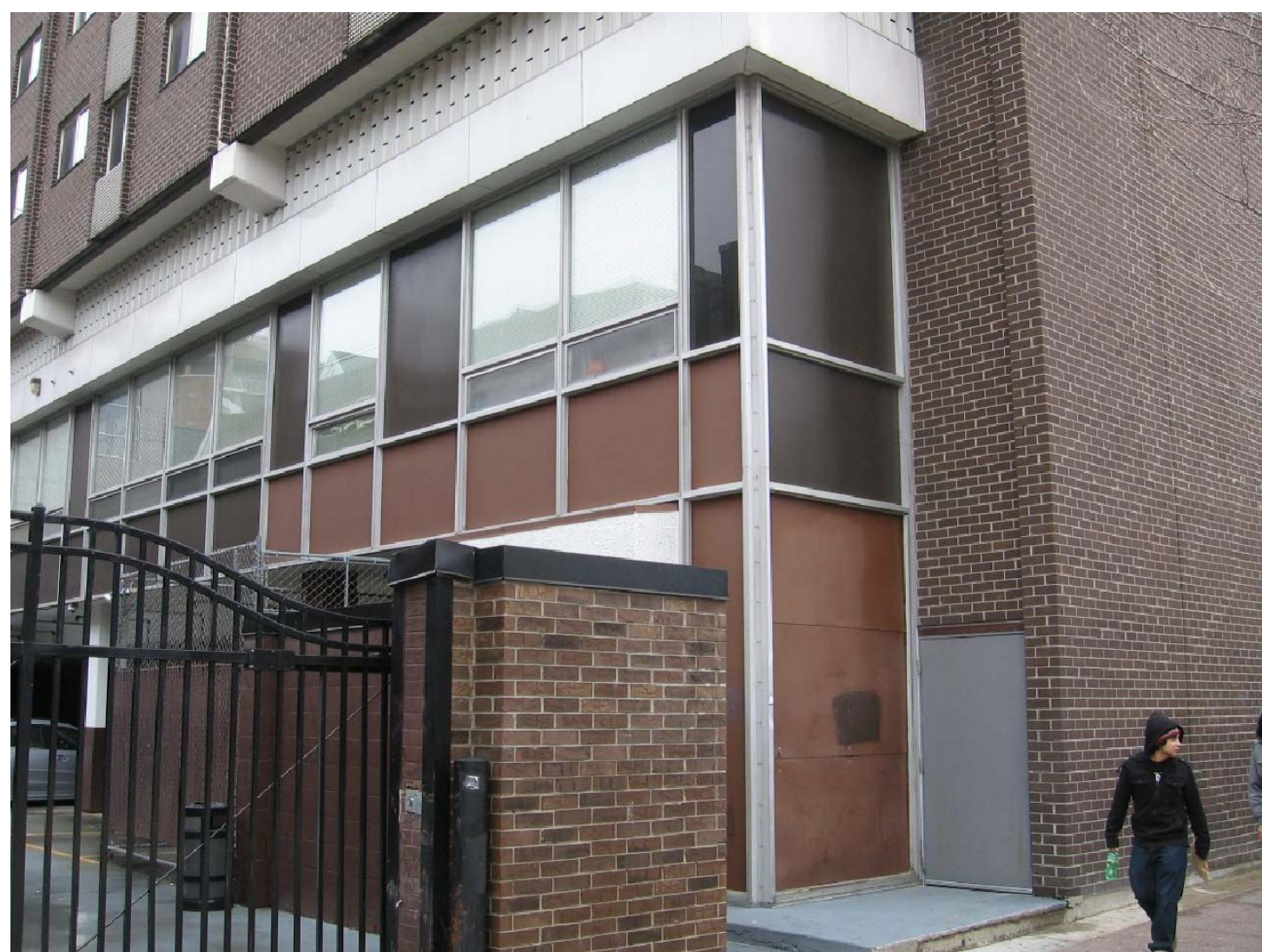
EXIT FROM EGRESS STAIR
