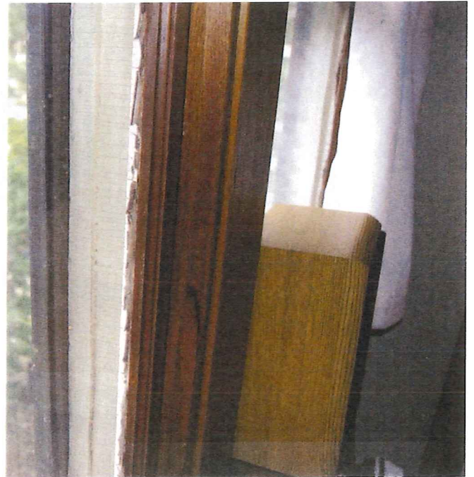
Glazing Failing
