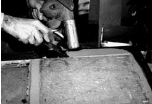
Sash can be removed and repaired in a convenient work area. Paint is being removed from this sash with a hot air gun. Photo: NPS files.
