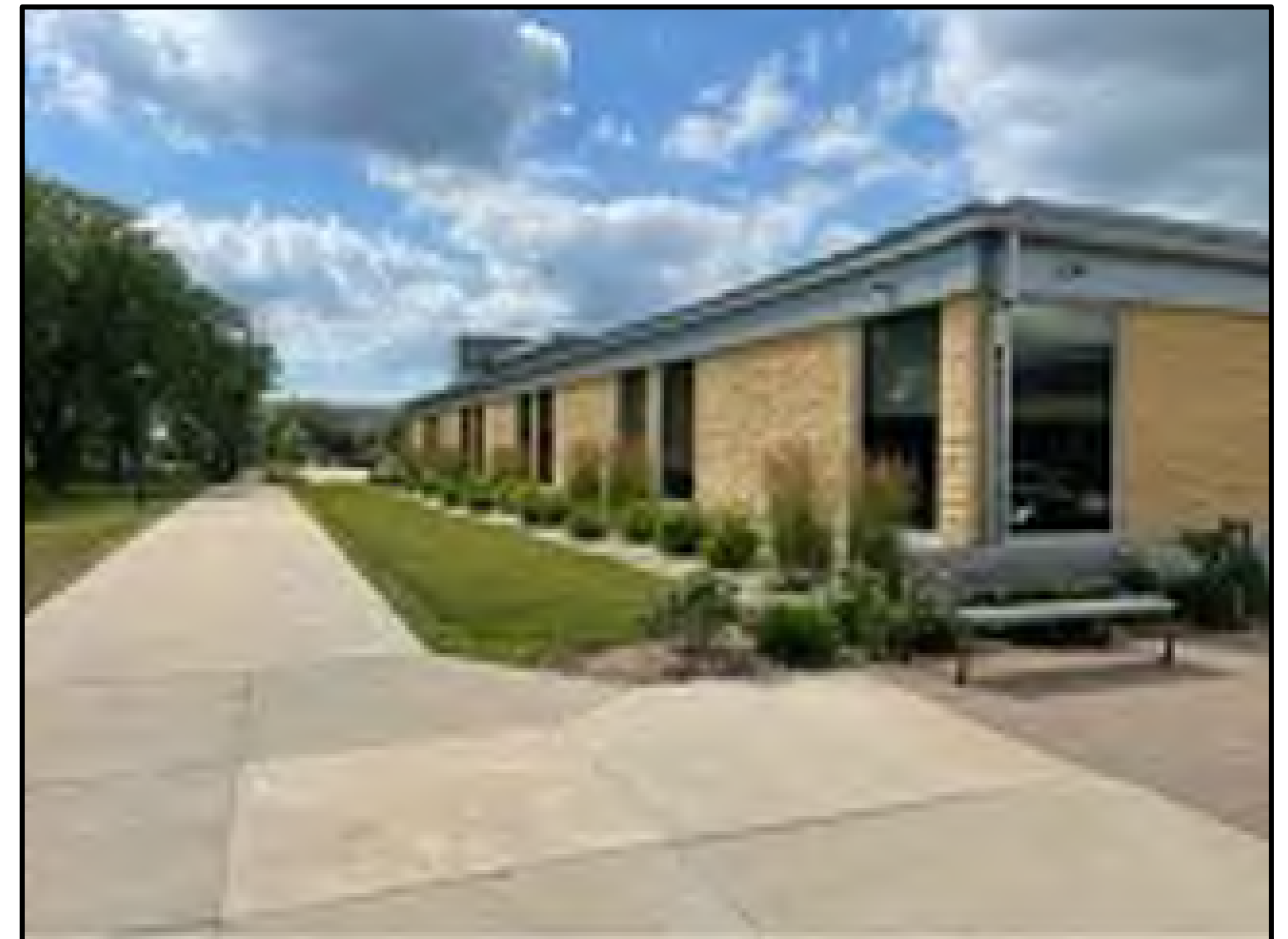
ADMINISTRATION BUILDING AREA
