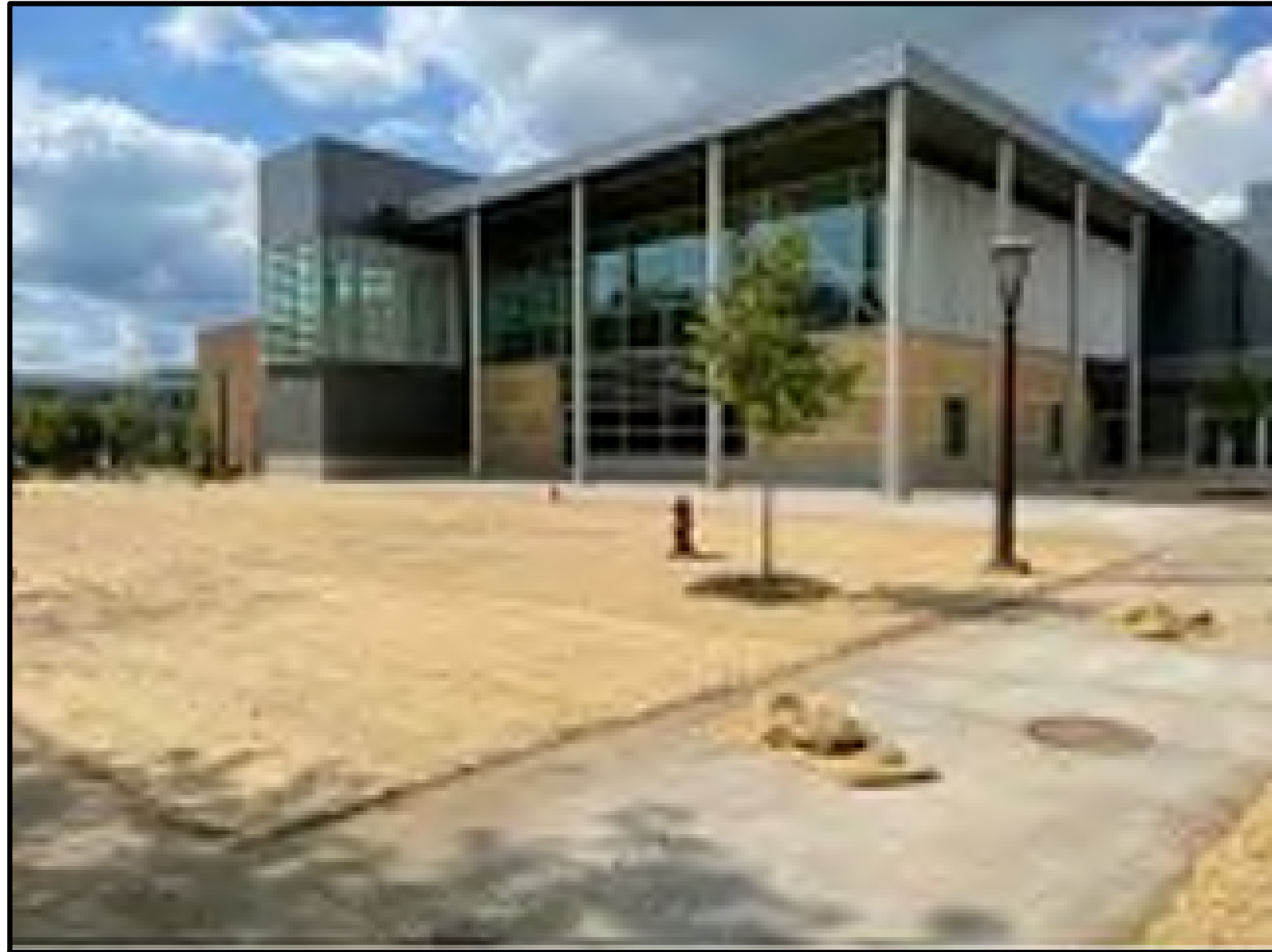
RECENT ADJACENT POOL AND FITNESS BUILDING AREA IMPROVEMENT
