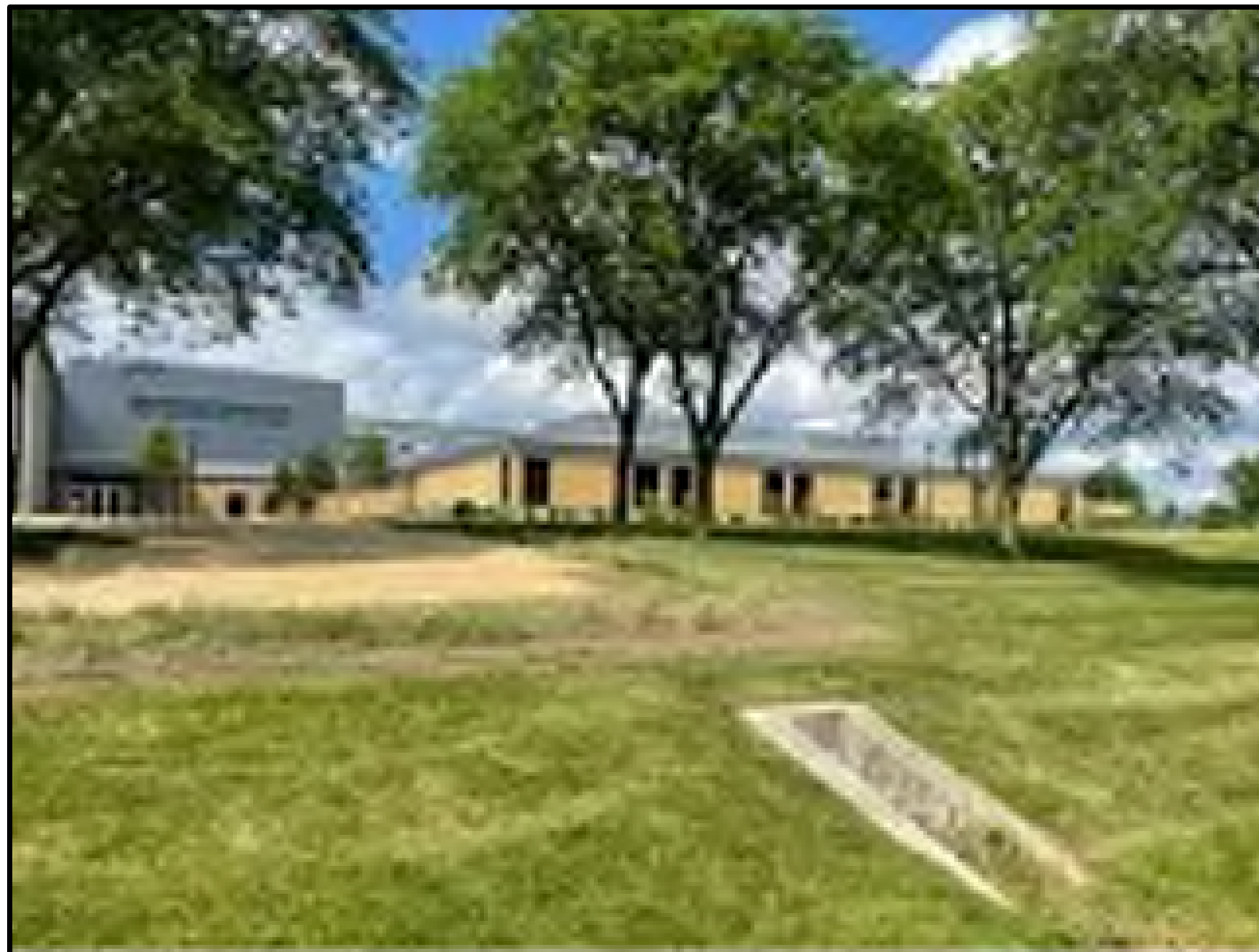
ADMINISTRATION BUILDING AREA
