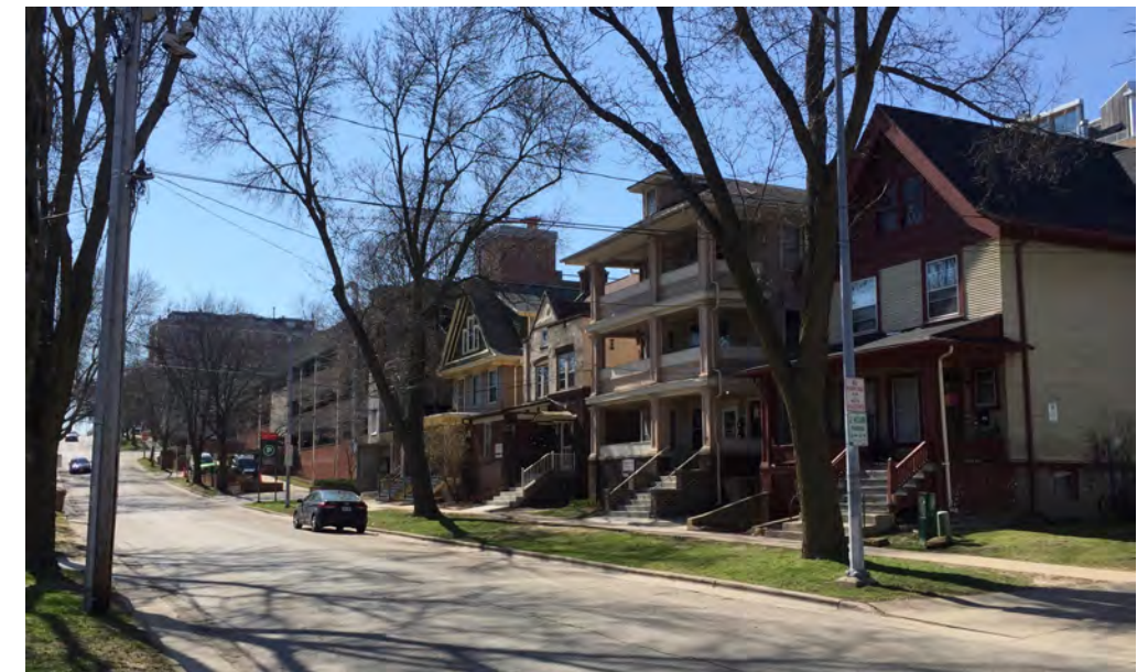
100 Block of North Butler looking Southwest
