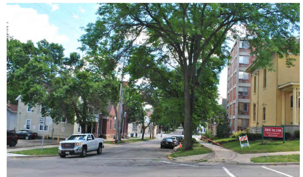
300 Block of North Butler looking Southwest
