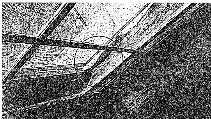
visible leaking on still and cracked and wood rot to storm window.
