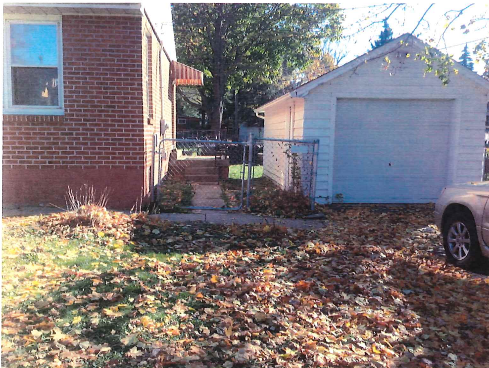
Front of existing garage
