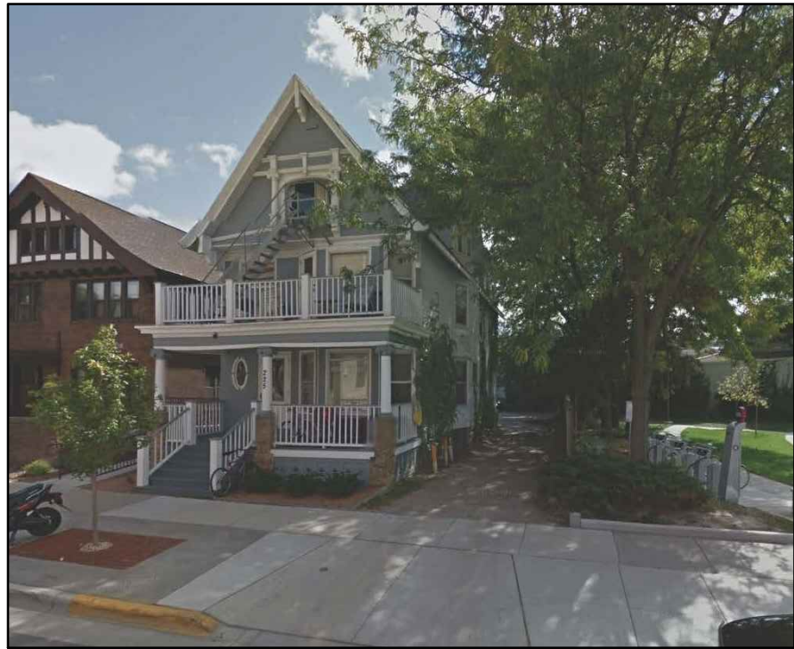
EXISTING BUILDING AND PARK ON GILMAN
