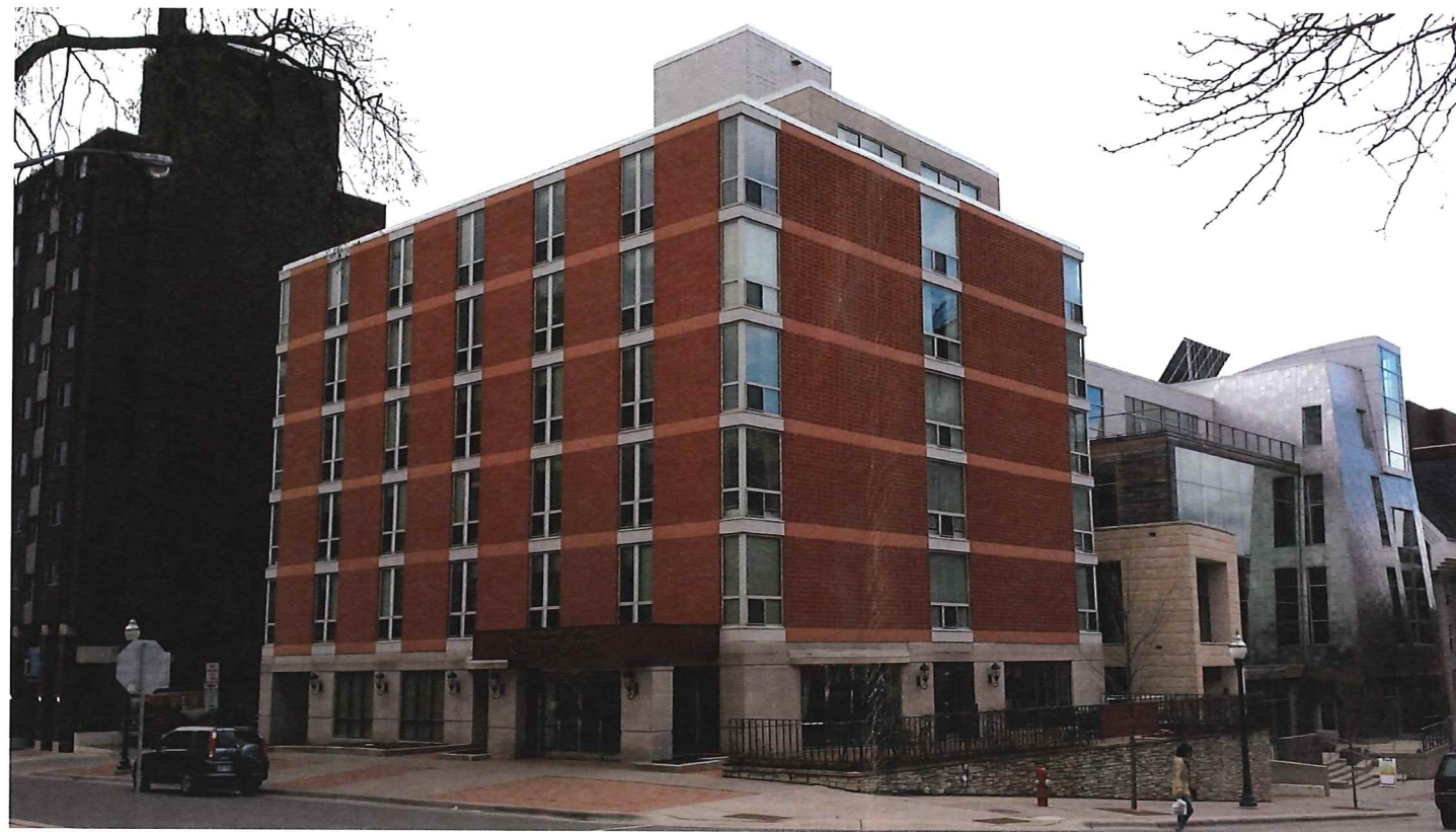
② EXISTING CONDITION
