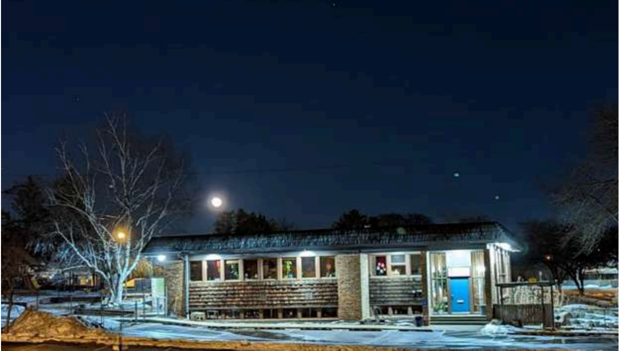
View from the parking lot of the proposed demolition site (5534 Medical Circle) towards the school (5530 Medical Circle)
