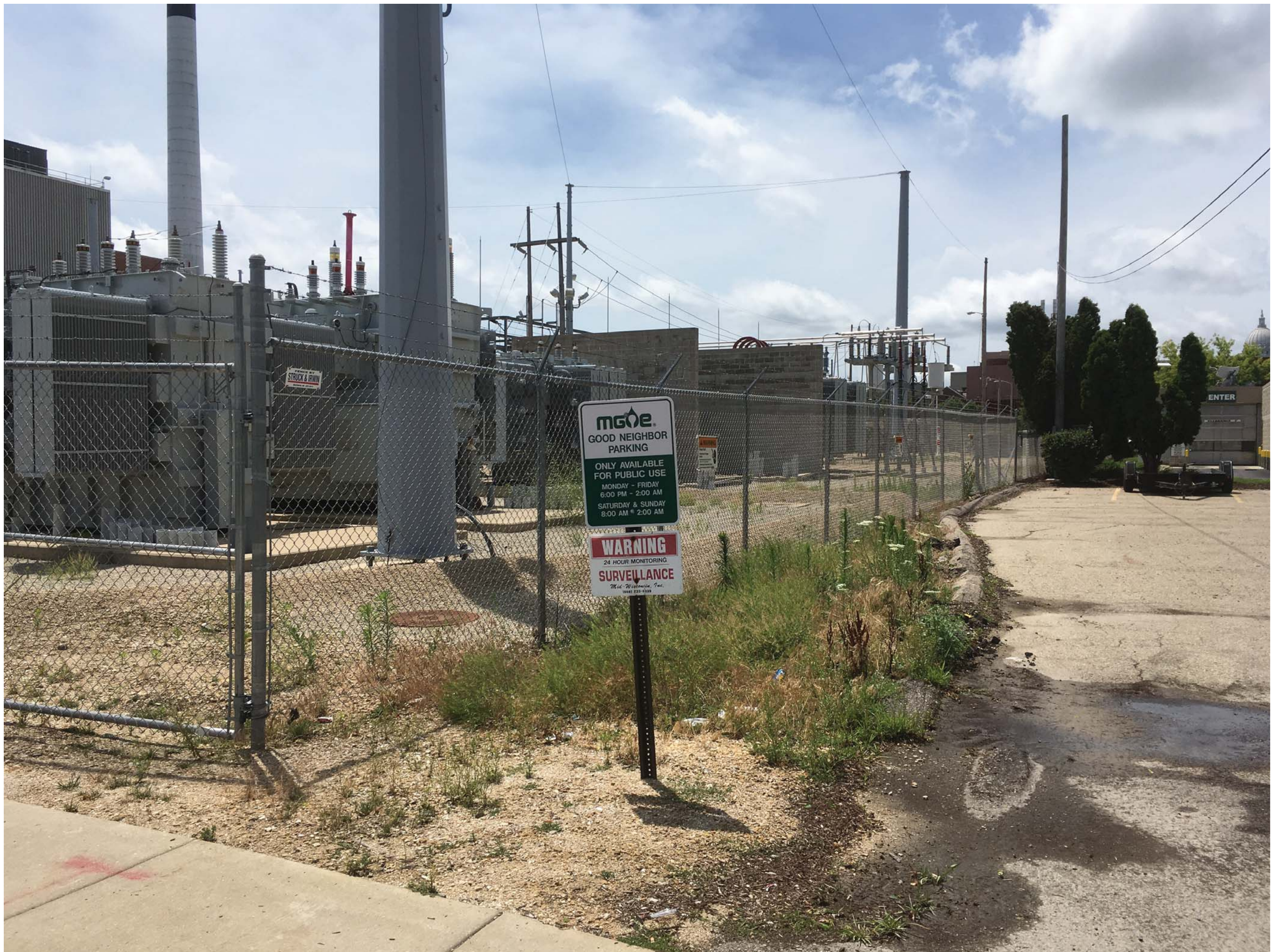
Northwest View - Facing East Washington Ave (Before)
